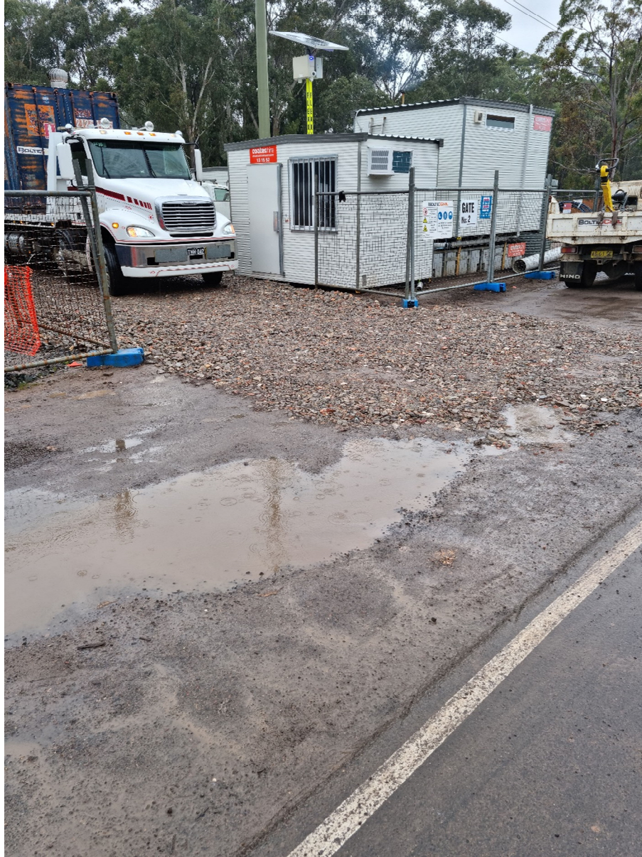
Site compound. Note the stabilised entrance/exit
