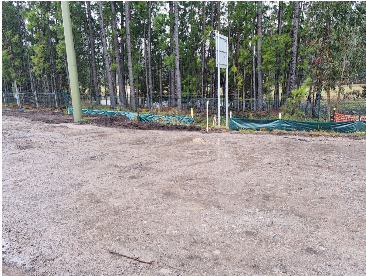
Erosion and sediment controls. Note the boundary exclusion fencing
