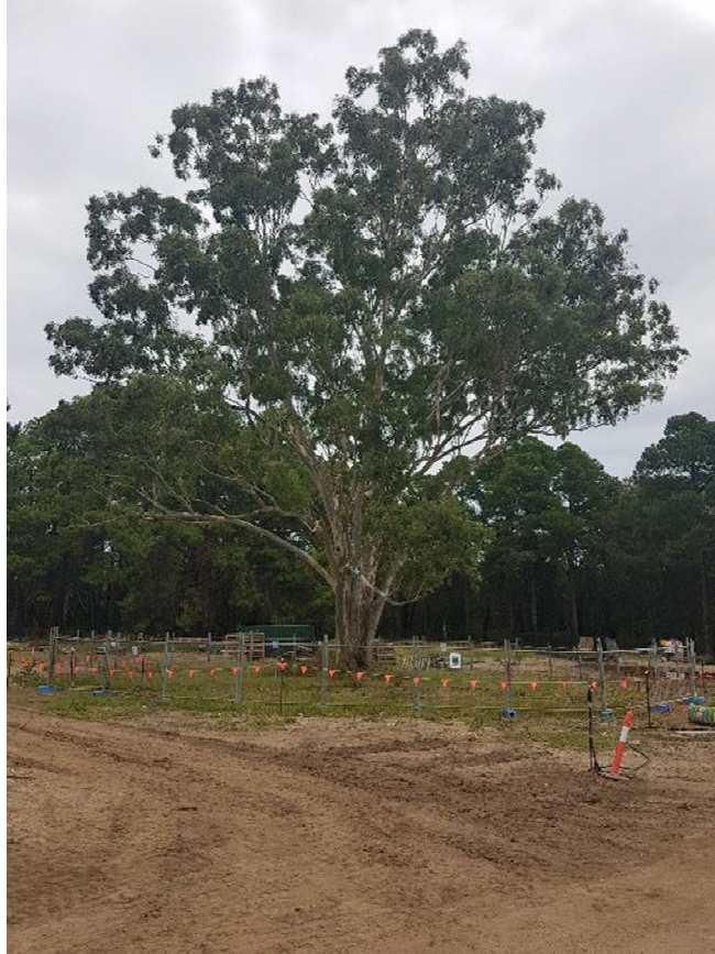
Tree protection measures in place
