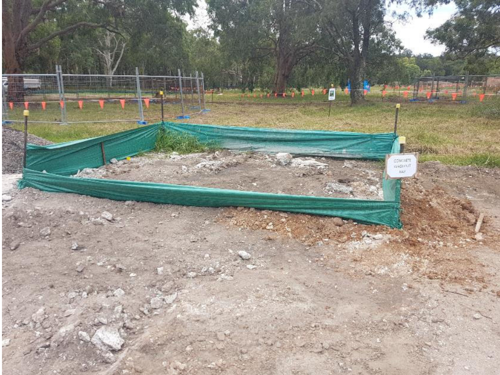
Concrete washout bay which needs rectification
