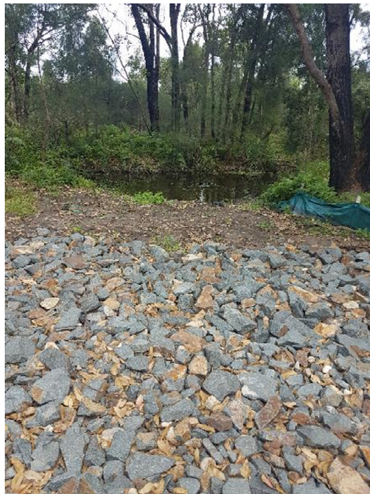
One of the completed stormwater discharge points
