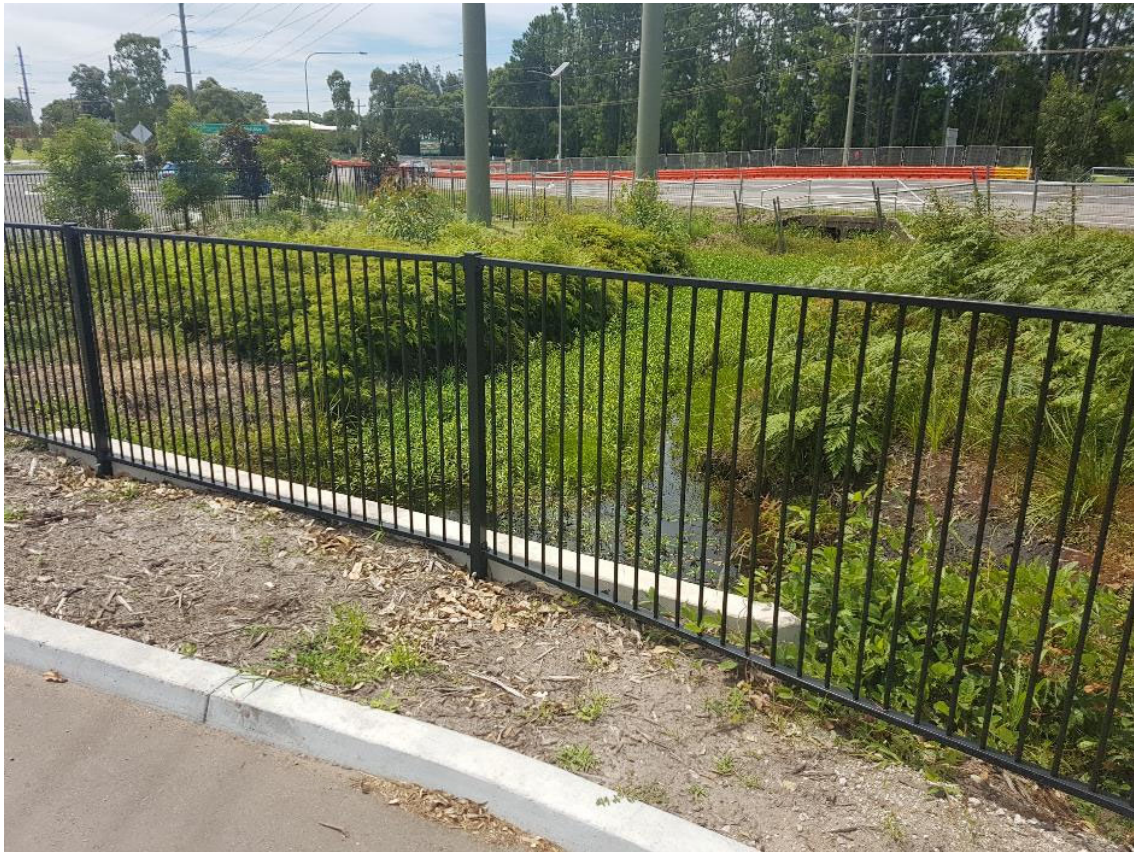
One of the completed stormwater discharge points
