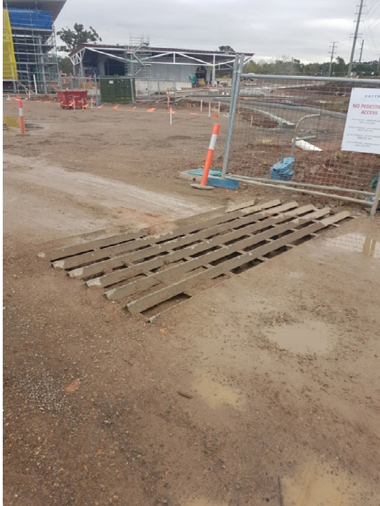
Shaker grid and wheel washing bay
