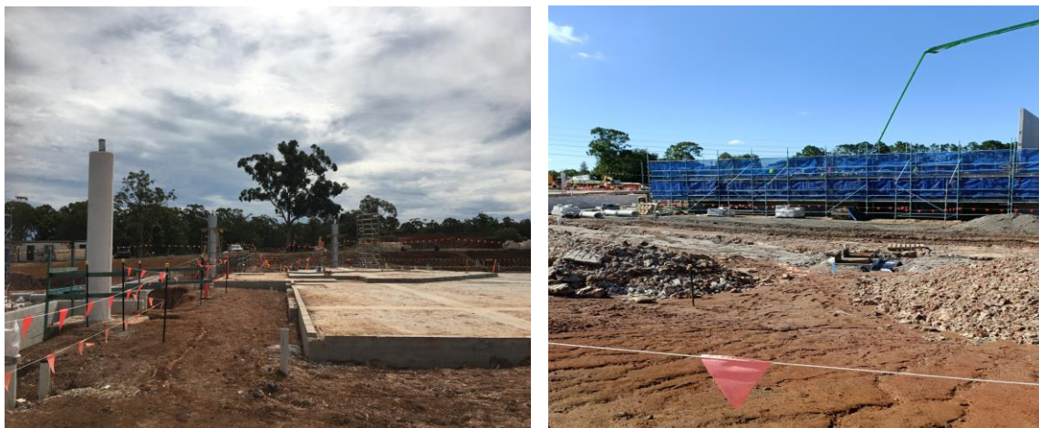
Photo 1 – Existing works on site
