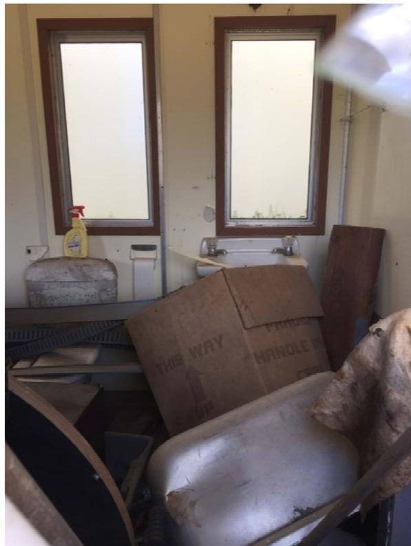
**PHOTOGRAPH 12** *Interior of the southern demountable which was primarily constructed of Masonite and laminate.*
