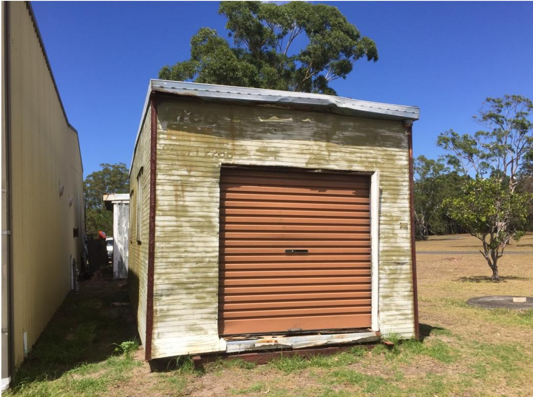
**PHOTOGRAPH 15** Exterior of the northern demountable which was painted metal (weathered).
