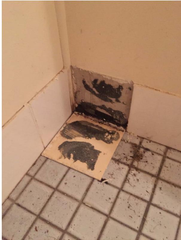
**PHOTOGRAPH 21** Ceramic tiles and underlying cement sheeting located within the toilet and bathroom in the shed that is considered to be the same material as Photographs 19 and 20.
