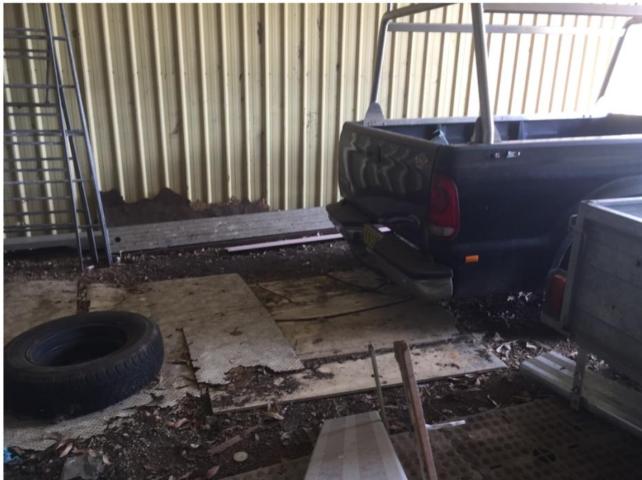
**PHOTOGRAPH 18** Materials being used to the line the dirt included masonite boards, rubber matting and fibrous concrete. One (1) bulk sample was collected for the asbestos identification in from the fibrous concrete which did not indicate the presence of asbestos.
