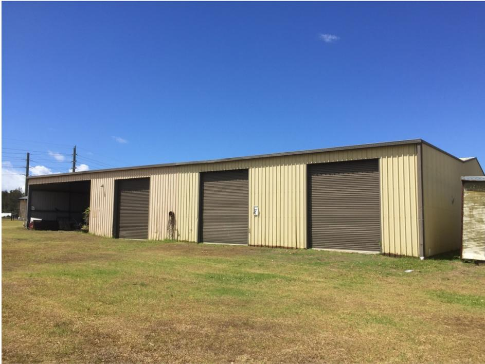
**PHOTOGRAPH 17** Northern aspect of the steel industrial sized shed. The far left portion (open door) was the only portion which was not underlain with concrete hardstand.
