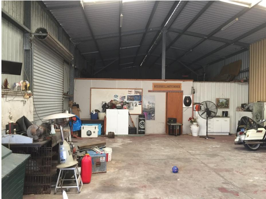
**PHOTOGRAPH 19** Interior of the shed (south eastern section). Construction materials included concrete floor, steel walls, roof and door. The shed was segregated into different areas using cement sheeting.
