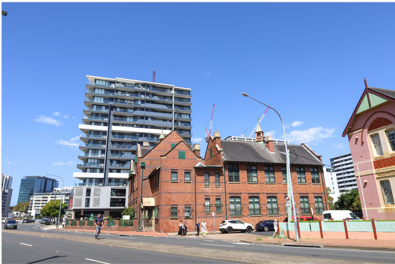
Existing site photo - Hannell Street
