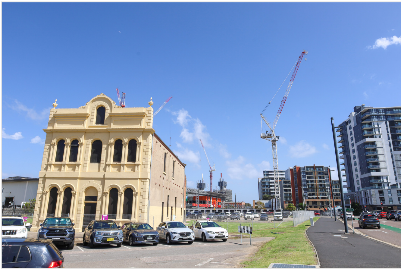
Existing site photo - Honeysuckle Drive
