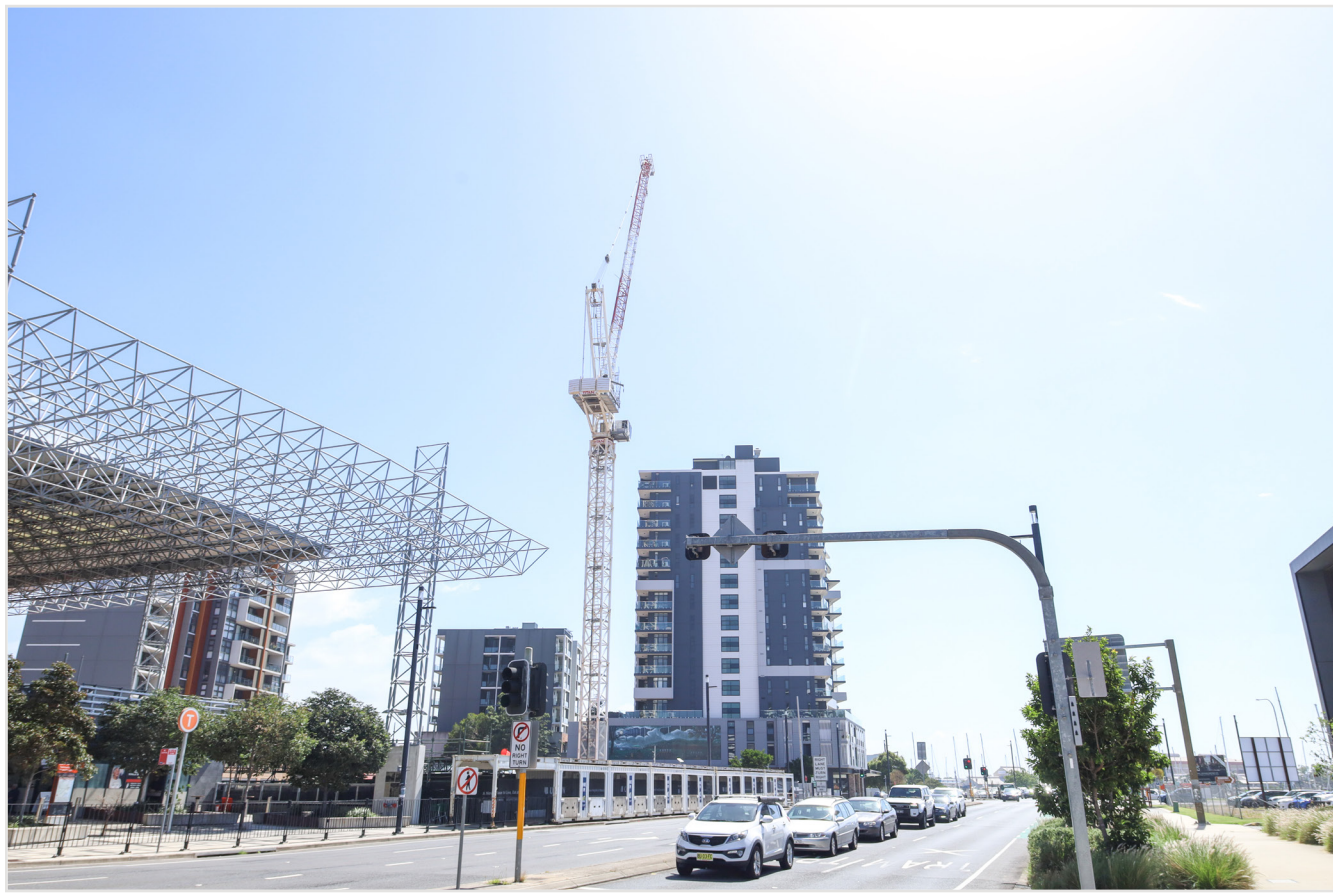
Existing site photo - Hannell Street
