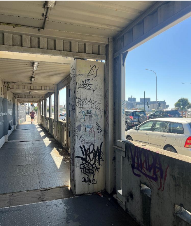
Graffiti, Hannell Street pedestrian walkway, looking northeast
