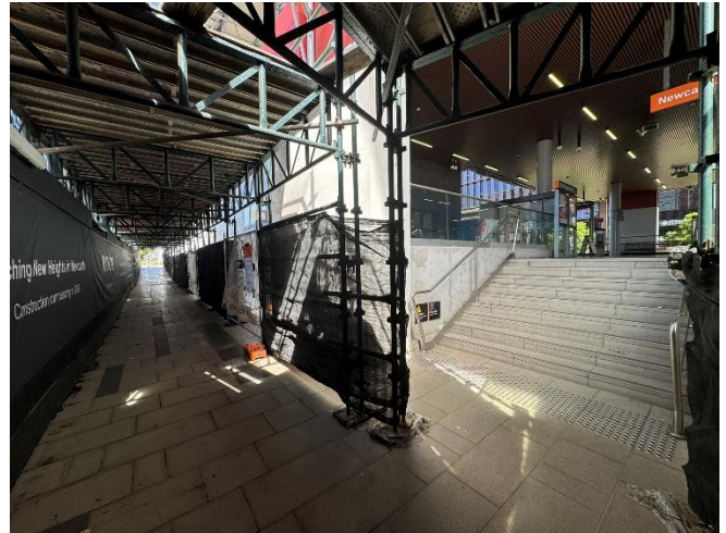
Temporary through-site link and stairs to Newcastle Interchange, looking southeast
