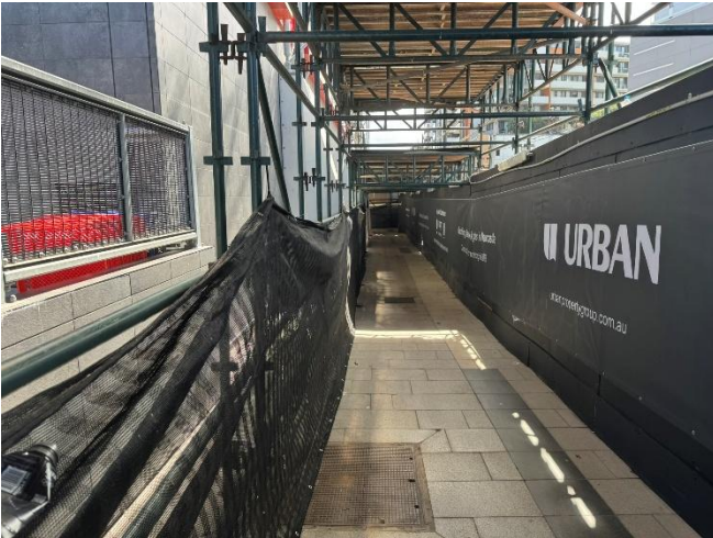
Temporary through-site link, looking west
