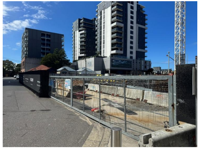
The site, western access point and Stella Apartments, looking northeast
