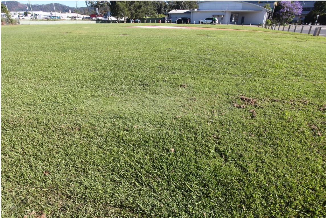
Figure 4: Raised grass are behind Ambulance Station (Helipad).
