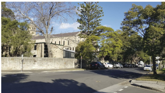
VIEW LOOKING SOUTH EAST FROM MARY ST (IMAGE PROVIDED BY ROBERTS DAY)
