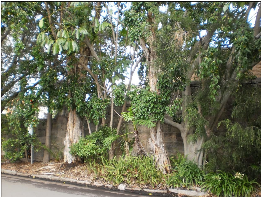
Photo F: Trees 33-35. These trees have the potential to damage the heritage sandstone wall.
