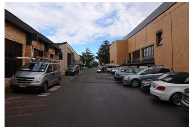
View looking east with Brother Emilian Hall on the right and underutilised buildings on the left to be demolished
