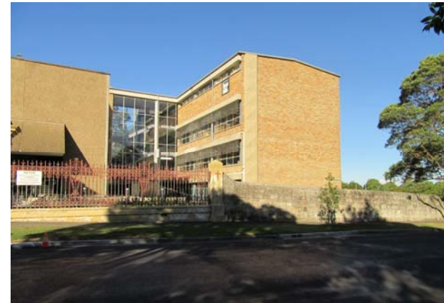
View looking south from Mary Street towards the 4 storey classroom building
