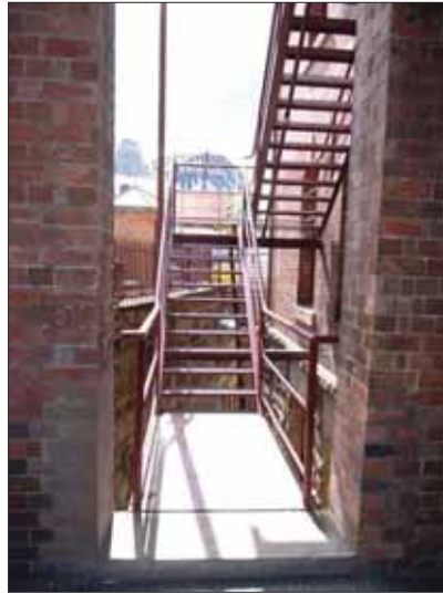
Figure 72: 1961 external fire stairs have been refurbished with a new opening from an original window at entry to the office block (Bay 1)
