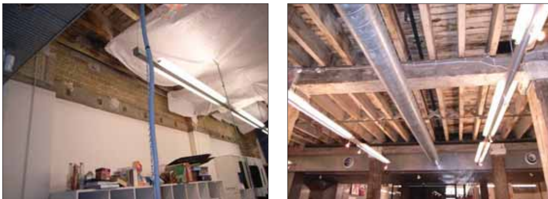
Figure 98: Views of the timber joists and underside of timber floor boards in Bay 4 of the third level. The suspended cloth ceiling is for temporary measures to protect from any dust caused due to the refurbishment works on the forth floor above. Note evidence of removed earlier suspended ceiling above the wall render of the left image
