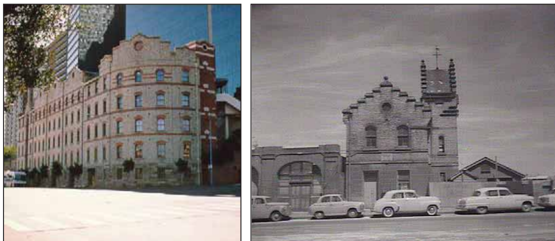
Figure 108: (Left) The Grafton Bond Complex, (now partly demolished) (Right) part of the office block at 1 Sussex Street, once part of the complex (Source: Left image, Graham Brooks & Assoc CMP, 2004. Right image, Mitchell Library Small Picture File)
