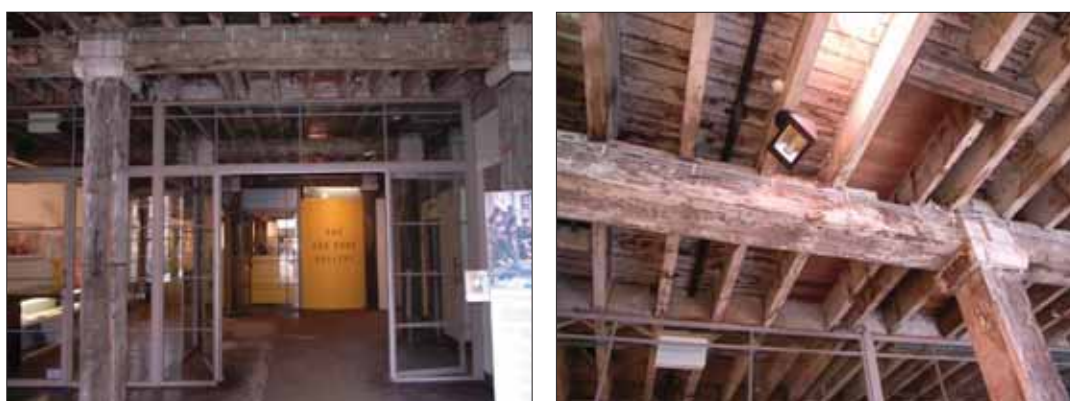
Figure 90: Entrance foyer to Bay 4 looking towards Ken Done Gallery and the lift foyer. Note terrazzo flooring to the foreground, and exposed timber ceiling structure (post and beam with cast iron capital) with evidence of repair and new services
