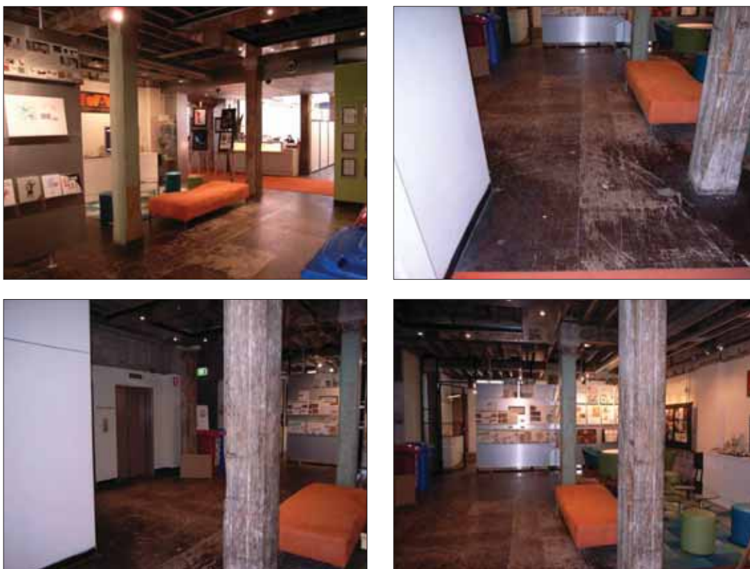
Figure 99: General views of warehouse Bays 2, 3 and 4 showing the concrete floor with asphalt finish and evidence of earlier uses trough marks on the floor
