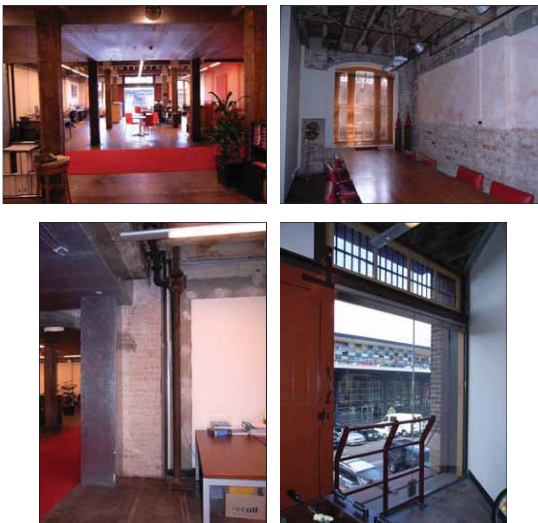
Figure 88: General views of Bays 2 to 4 showing air-condition ducts along the centre corridor between the arched openings, remnant rendered and painted wall of the 1950s-1960s alterations with original facebrick walls partially exposed, original fire services downpipe and the new glass insertions to loading doors with metal safety barriers.
