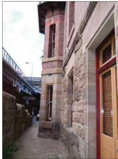
Figure 75: (Far left top) Ground floor level of the office block with rockfaced ashlar stone walls and retaining wall below Hickson Road, external toilets are behind the iron grille gate, which appears to have an access door to the warehouse bay beyond, now kept closed. 1961 fire stairs are above.
