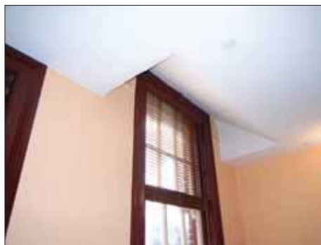
Figure 101: Bay 1 office block showing western office space (top), timber stair to clearstorey (centre) during restoration in 1990s and in 2008 with clearstorey above, western amenities with early tiles, and detail of pitched lath and plaster ceiling to form dormer windows
