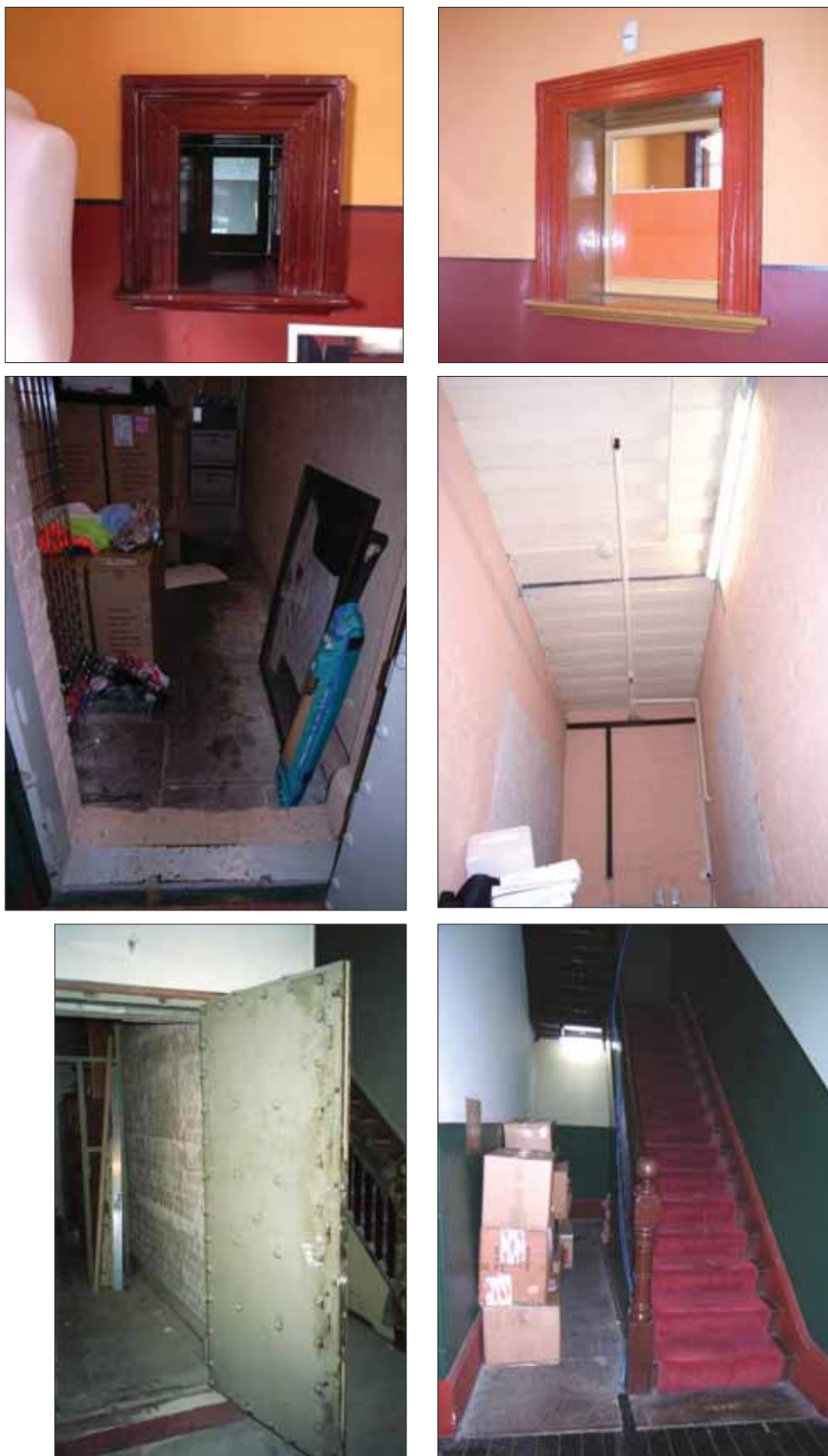
Figure 97: Service and communication windows, safe room with flagstone floors and timber board ceiling, safe during restorations, and restored original timber stair (Source for 1990s image the Foreshore Authority)
