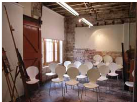
Figure 99: Above left is the view of Bay 4 looking west towards the lift foyer, above views through the original arched openings with air-conditioning duct in between, the classroom on the left facing the George Street elevation and features layers of finishes from the original to the 1950s-1960s and reconstructed loading doors. The top sash rail of the timber window seen here is partially broken and requires repair in splicing form.
