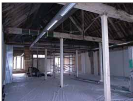
Figure 103: The fourth floor warehouse bays with Kingpost trusses and beams, sawtooth gabled roof form, timber rafters, brick gable ends, arched loading doors with louvered tops, glazed transoms and timber board doors. New light fittings and services and carpet flooring are for the new tenancy fit-out. Note original fire sprinklers under the roof lining
