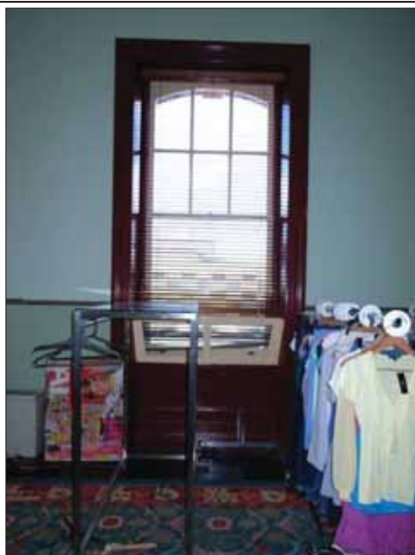
Figure 95: Example of reconstructed timber framed sash window with two mullions and other retained and reinstated features of Bay 1: fireplaces and overall office fabric/joinery.
