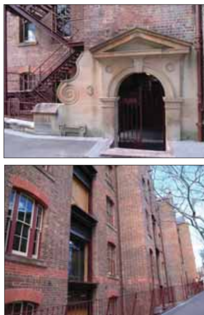
Figure 74: (Far left) south most end of Bay 5 showing overall gable detailing including round accent window, arched loading bay with restored pulley and cathead, segmental arched window openings with stone sills, copper rainwater head and downpipe, and original bracket that was used for supporting the overhead wires for trams at 3 rd floor window lintel level (Left top) decorative dressed stone entrance to office block with classical motifs and scrolls (Left bottom) warehouse bays showing the stepping articulation of the bays from Hickson Road to George Street
