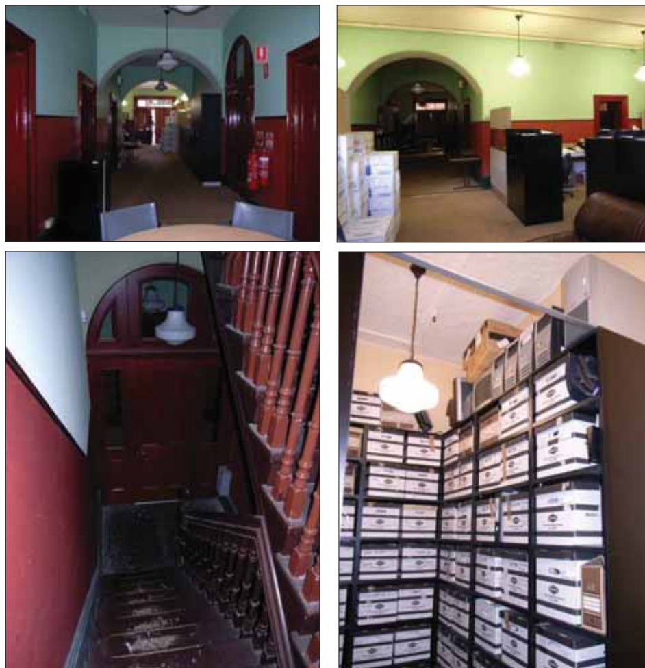
Figure 77: General views of Office block ground floor (Bay 1) showing main corridor, eastern office, worn timber stair and pressed metal ceiling
