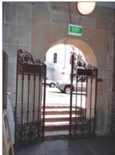
Figure 73: (Far left) original panelled timber entrance door with sidelights and transom window, and (Left) decorative wrought iron gates to the office block (Bay 1)
