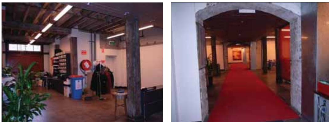
Figure 87: Bay 1 Warehouse component where McLachlar Lister Company occupies Bays 2 to 4. Left is the 1950s stairs in Bay 3 looking towards George Street, interconnected character of the bays and warehouse quality of the space are evident on the right image
