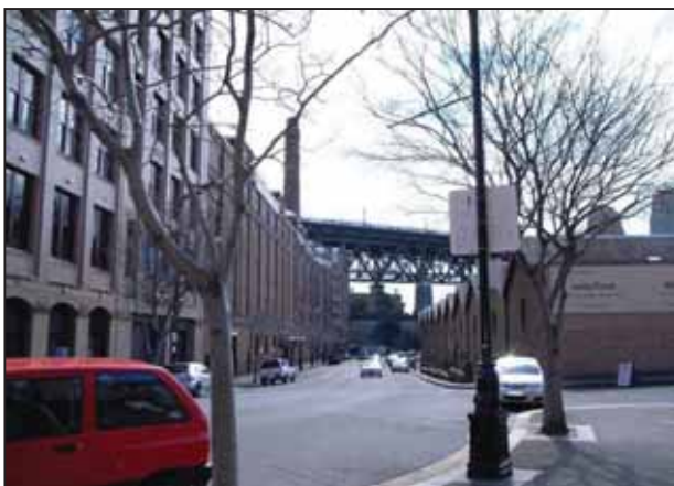
Figure 58: Looking north along Hickson Road to the Harbour Bridge approaches. The Metcalfe Bond Stores and former Mining Museum are on the left, Campbell's stores are on the right
