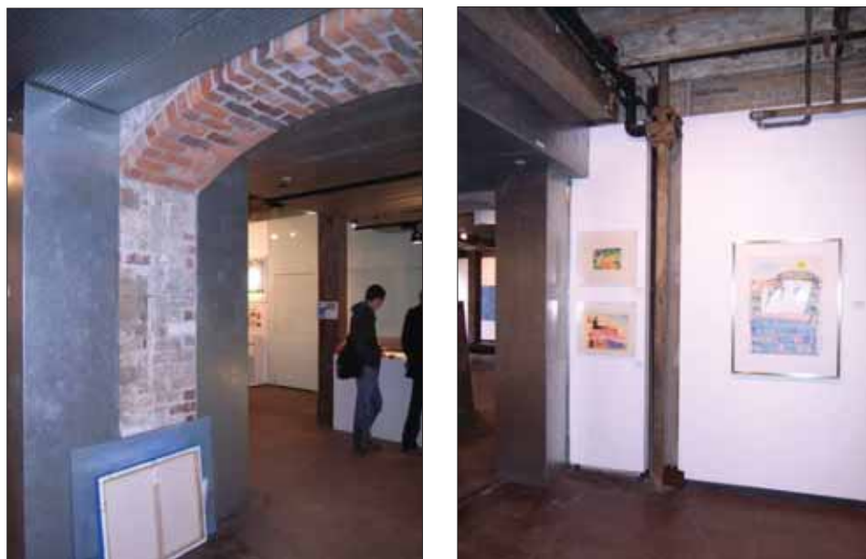
Figure 93: The Ken Done Gallery showing the repaired brick arch opening, and original fire services
