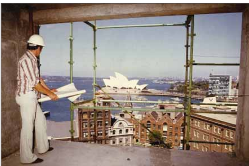
Figure 47: c.1970s photograph showing the ASN Co. Building at centre, called at this time, the Ordinance Stores, with Opera House at the background. Probably taken from the 1970s Sirius Apartments near Gloucester Walk. (Source: Foreshore Authority 38968_HIM_47)
