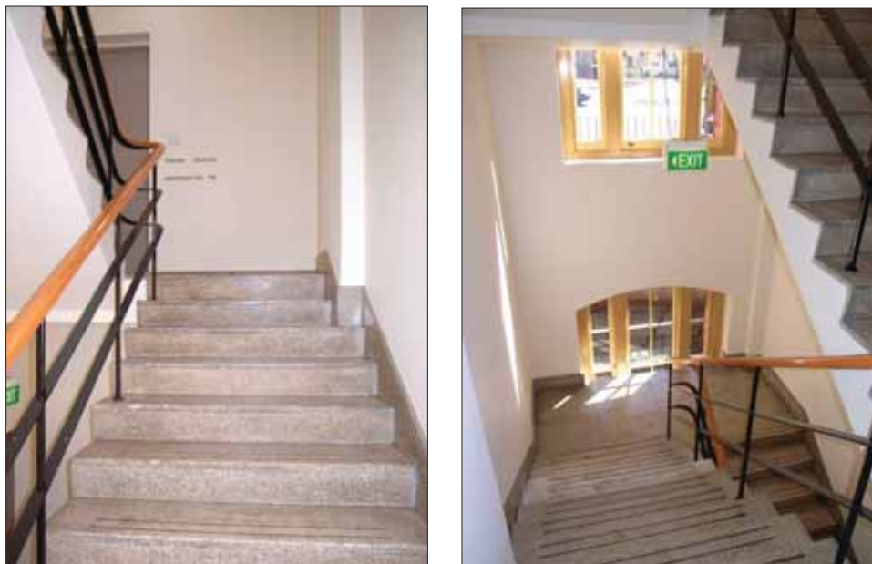
Figure 102: The 1950s firestairs on the south-western corner of Bay 4 featuring terrazzo steps, iron balustrade and timber hand railing. Note floor identification signage consistent throughout all building levels
