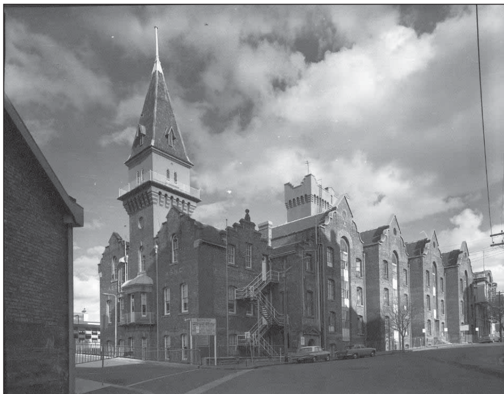
Figure 28: 1970 Photograph of the ASN Co. Building (Source: Sydney Harbour Foreshore Authority, 39971_A742-166)
