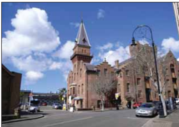
Figure 62: View of the former ASN Co. Building from George Street looking east with the Overseas Passenger Terminal in the background.
