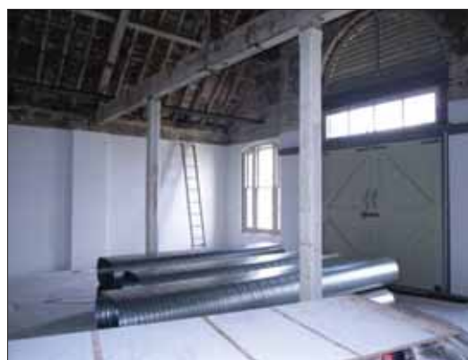
Figure 103: The fourth floor warehouse bays with Kingpost trusses and beams, sawtooth gabled roof form, timber rafters, brick gable ends, arched loading doors with louvered tops, glazed transoms and timber board doors. New light fittings and services and carpet flooring are for the new tenancy fit-out. Note original fire sprinklers under the roof lining
