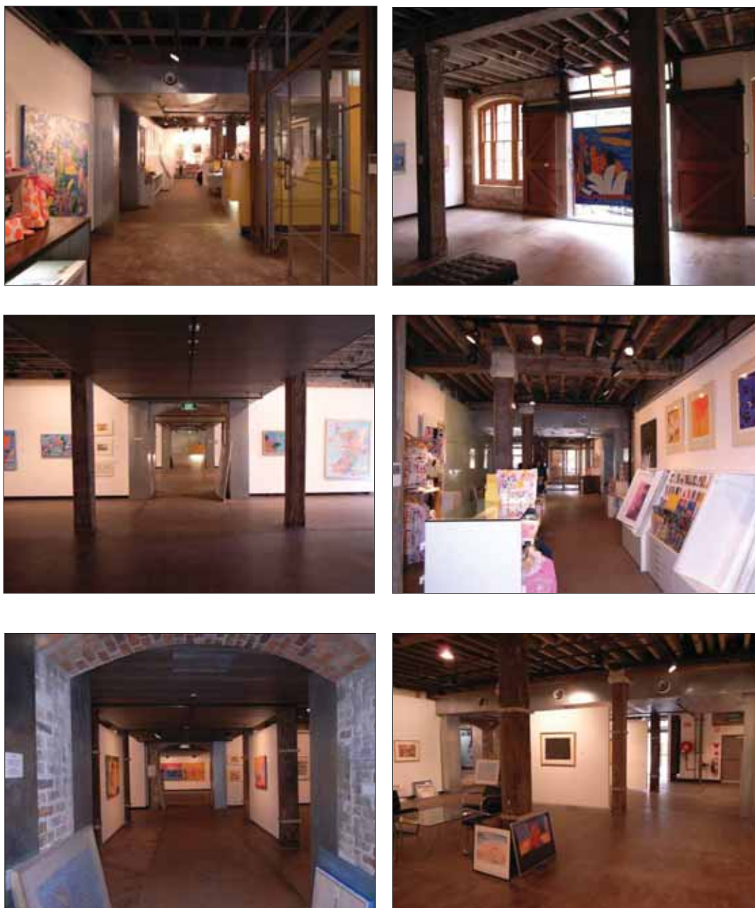
Figure 92: General views from the Ken Done Gallery showing the original open plan warehouse character and layout of the Bays 2, 3 and 4. Exposed timber ceiling structure and structural posts, new services including air-conditioning duct in the centre left image, glass and plasterboard partitions, and repaired brick arch opening. Use of the spaces as gallery maintains the opportunity for appreciation of the warehouse qualities of the former ASN Co. Building
