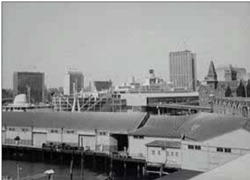
Figure 27: 1963 Overseas Passenger Terminal and Circular Quay looking from Dawes Point Park (Source: City of Sydney Archives, 013/0136171963)
