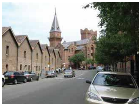
Figure 55: 1987 and 2007 views of the ASN Co. Building from Hickson Road.
