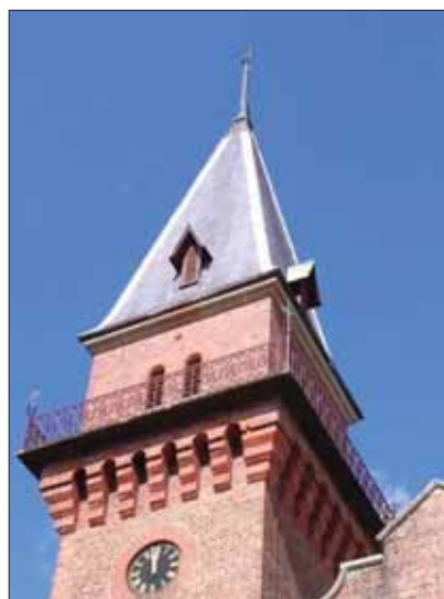
Figure 76: (Far left) original 12-pane timber framed windows to the top floor of office block (Bay 1) on eastern elevation, and (Left) clock tower with original louvered windows, and restored spire, iron balustrade and clock
