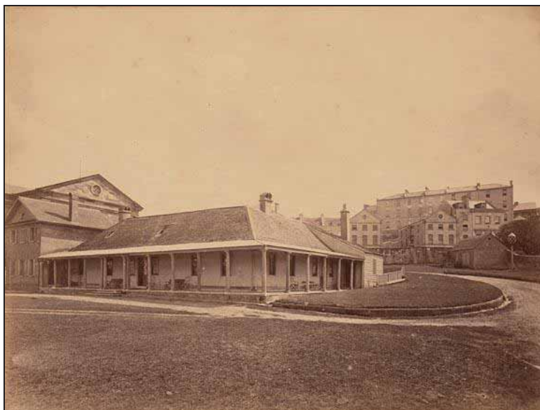
Figure 10: 1870s photograph of Campbells Wharf House. The ASN Co. occupied this house until it was demolished to reconstruct the ASN Co. Building. (Source: Mitchell Library, Small Picture File 350)
