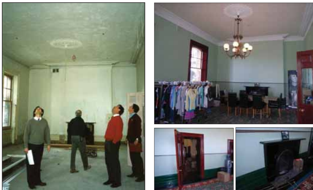
Figure 94: The eastern side office on the Second floor of Bay 1 showing the room during the 1990s restoration works and in 2008. Note new Victorian colour scheme, highlighted plaster moulded cornices, ceiling rose and slate fireplace (Source for 1990s image the Foreshore Authority)
