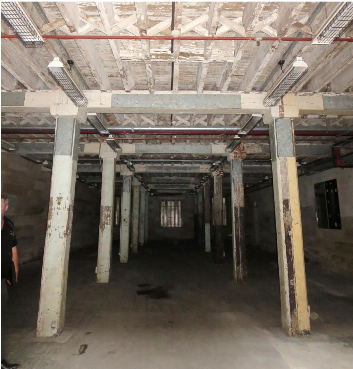
Figure 5: Internal photograph of Bay 5.
