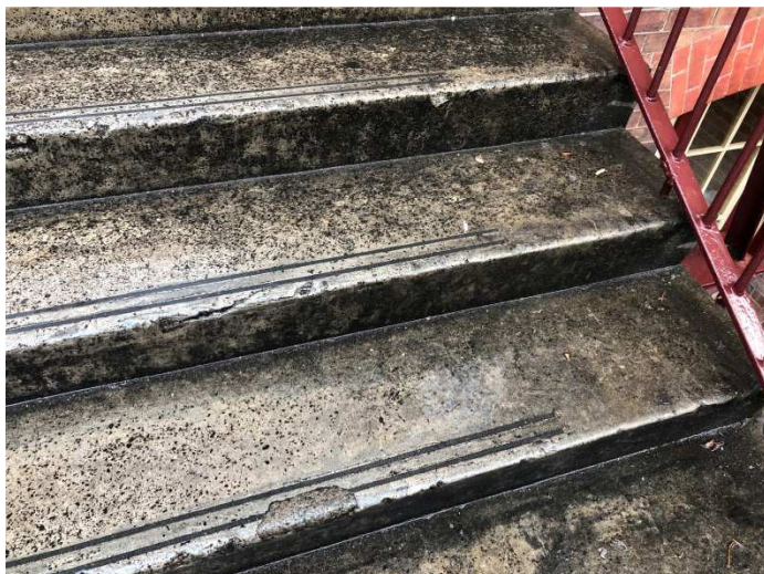
Steps 2 – after rain view
