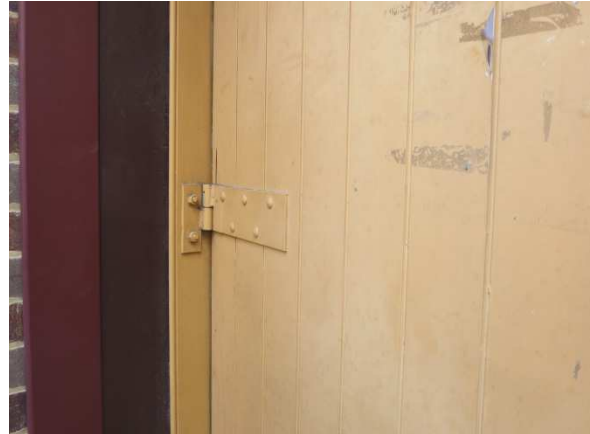
Level 2 Bay 5 Existing entry Door 5L2/XD1 Existing strap hinges to remain.
