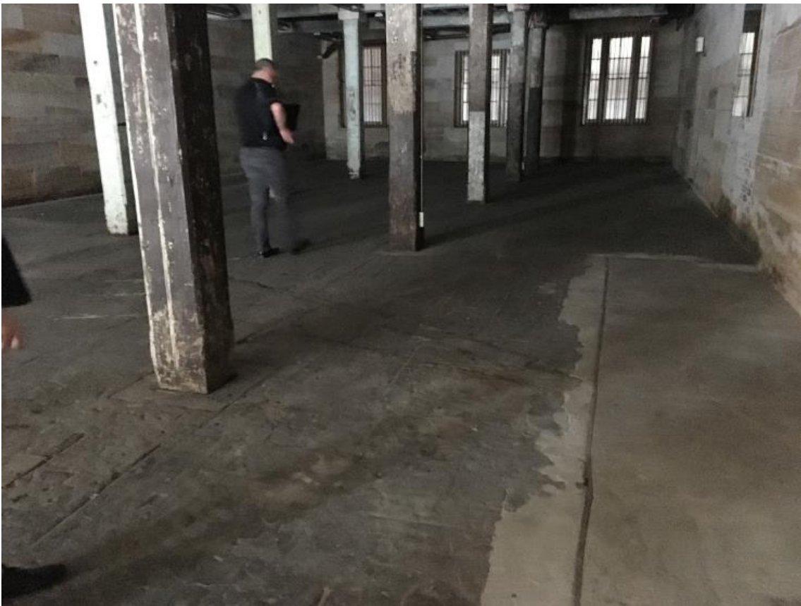
Figure 8: Looking west, showing the existing services trench running adjacent to north wall.
