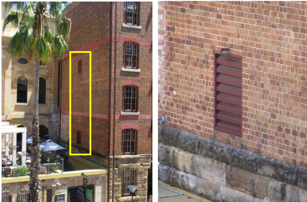
46 Early 1990s metal louvres in openings located on the southern elevation of the ASN Co Building.
