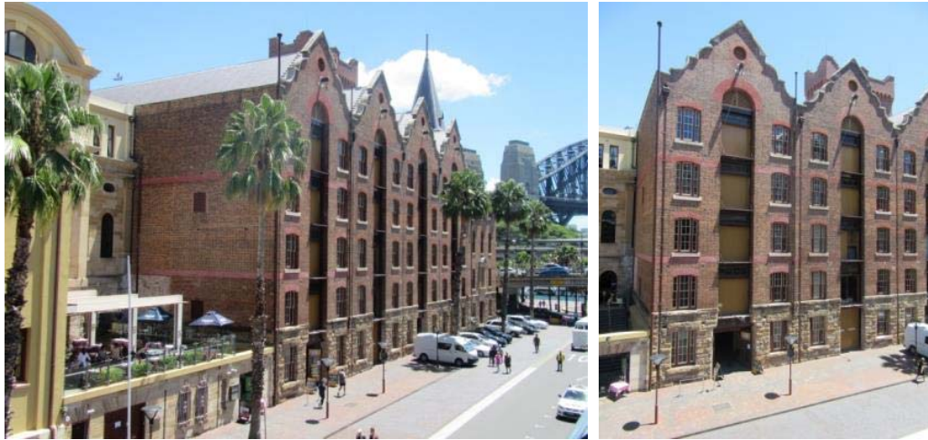
45 The ASN Co Building viewed from the south east (left); eastern façade of Bays 4 and 5 (right).
