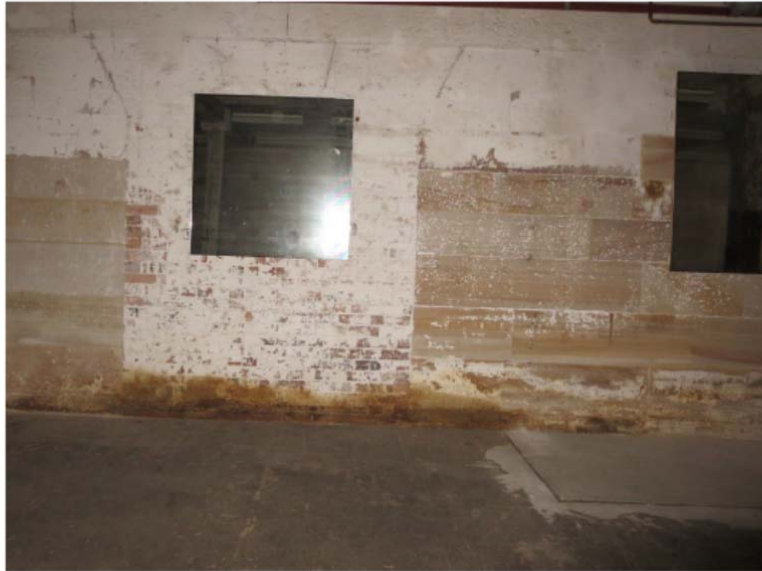
Figure 7: Looking north. The western end of the existing services trench is at right.
