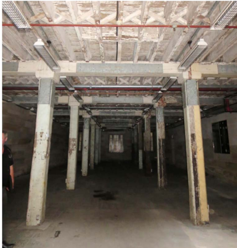
Figure 5: Internal photograph of Bay 5.
