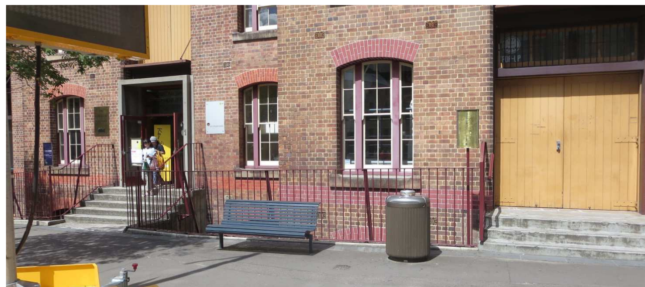
3. Closer view of the balustrade at the entries into Bays 4 and 5
