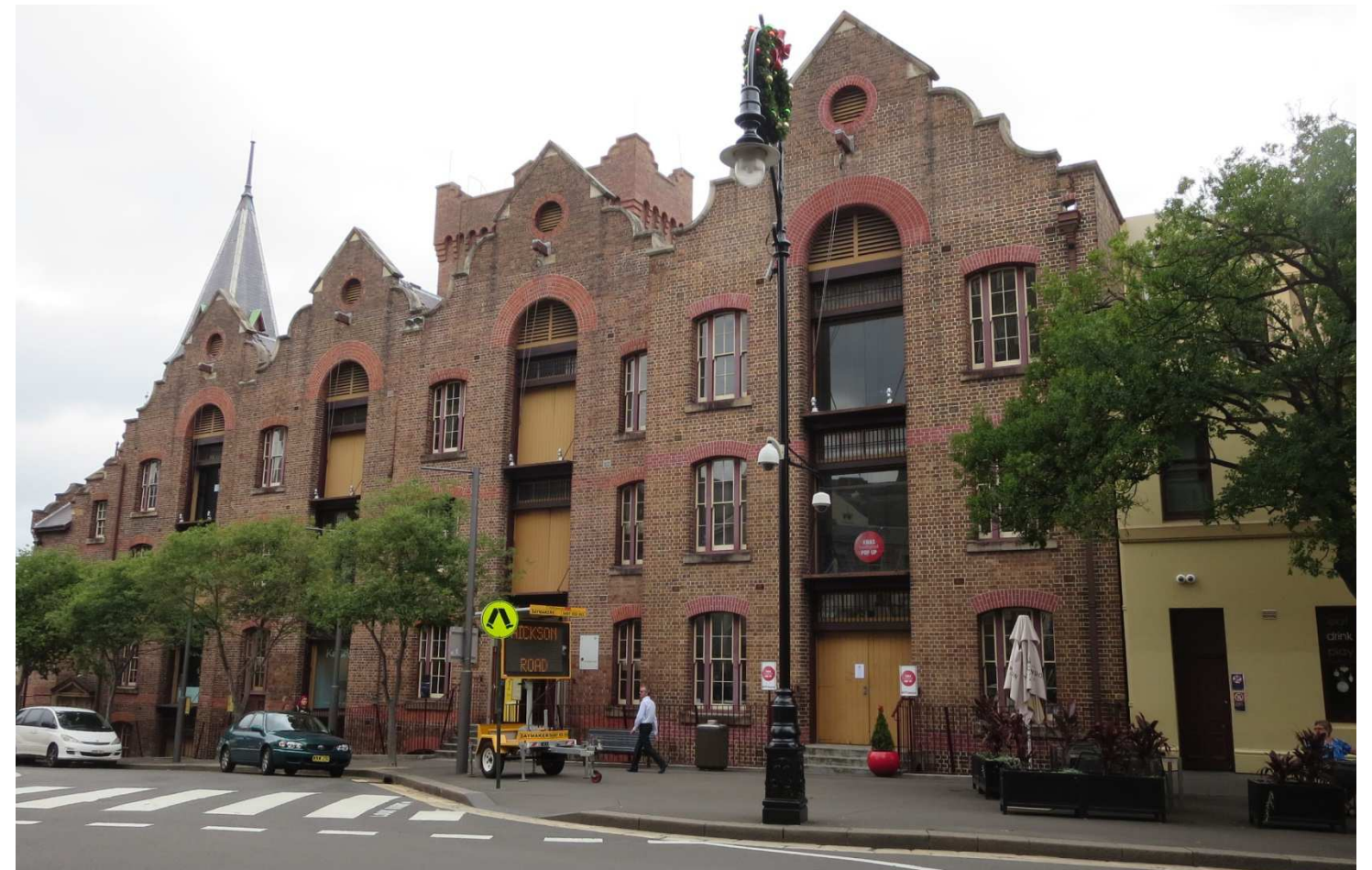
2. Existing view of ASN Building looking north east from George Street
