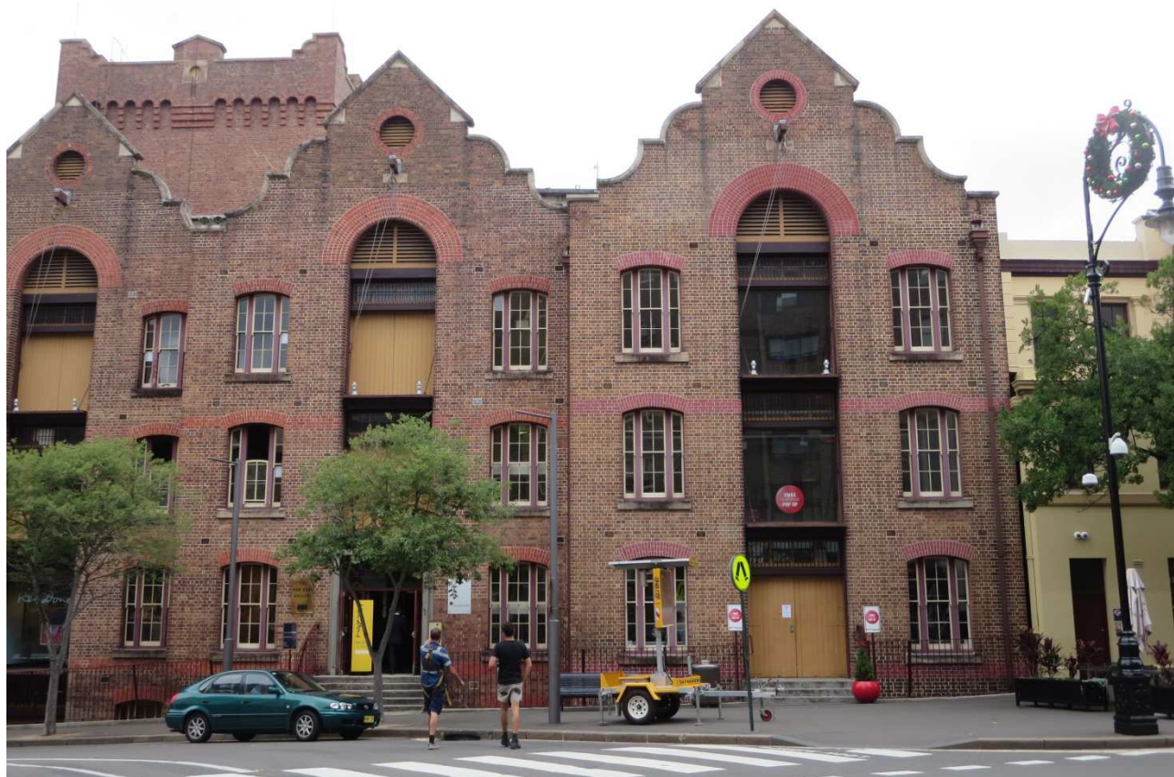
1. Existing view of entry into Bays 4 and 5 from across George Street
