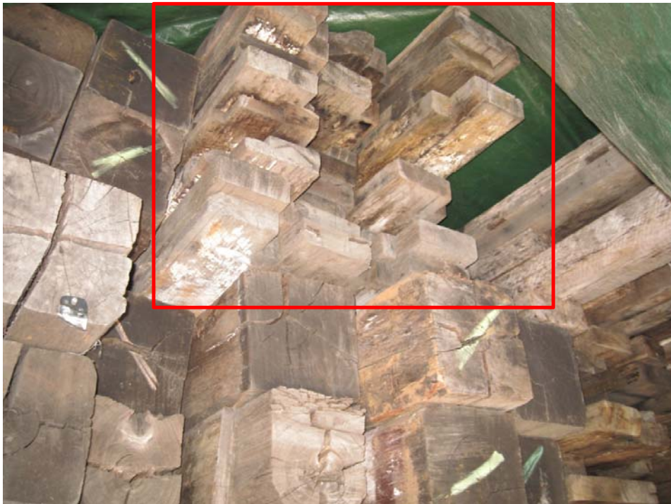
8. Packs of timber joists (shown in red box) located under tarpaulin. The other larger section timbers shown are additional beams or columns of various condition as noted in the summary above.
