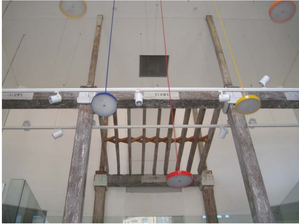
13. Example timber construction remaining insitu at 5 Hickson Road, The Rocks. Level 3 and 4.
