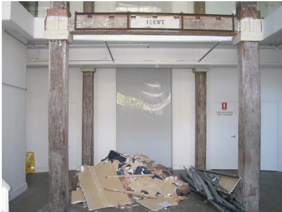
14. Example timber construction remaining insitu at 5 Hickson Road, The Rocks. Level 2.
