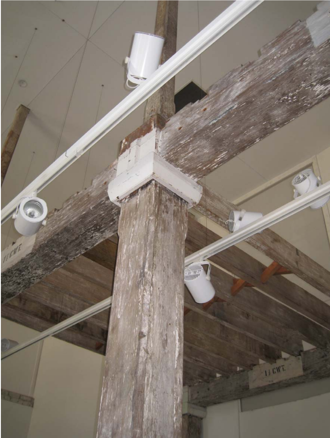
19. Example of timber construction detail remaining insitu at 5 Hickson Road, The Rocks.
