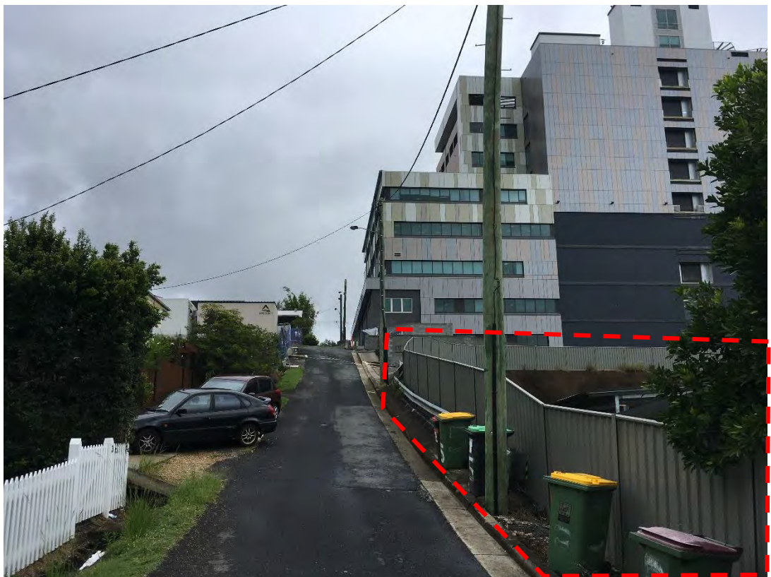
Figure 9: The location of the proposed works is to the rear of the southern tower (outlined in red). There is currently no development present on the site. (Source: courtesy of John Holland)
