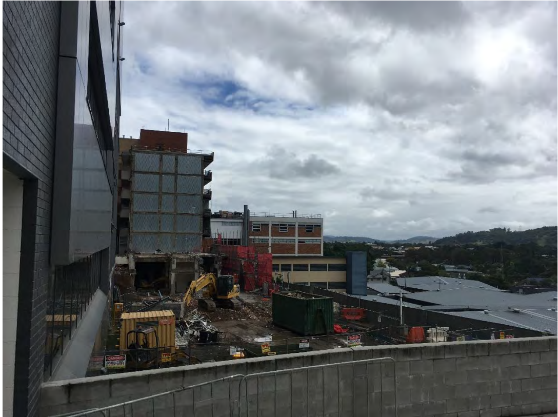
Figure 10: The site of the soon to be constructed northern tower.
