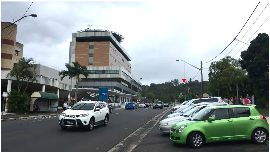
Figure 14: View 1 looking east from within Uralba Street. The heritage item is not readily visible due to existing street landscaping. While landscaping is not a permanent feature, this view is not considered of significance.
