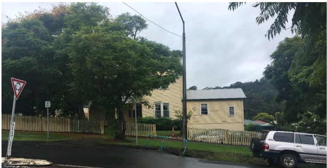
Figure 22: View of the heritage item looking east from within Dibbs Street.
