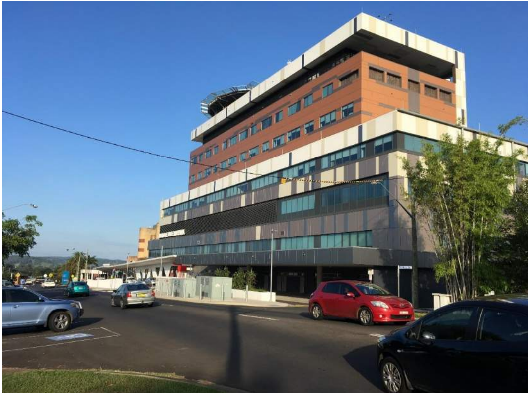
Figure 9 View of the south-eastern corner of LBH with the newly constructed Stage 3A building in the forefront. The proposed NTX tower will be constructed to the north/behind Stage 3A (Source: JHG)
