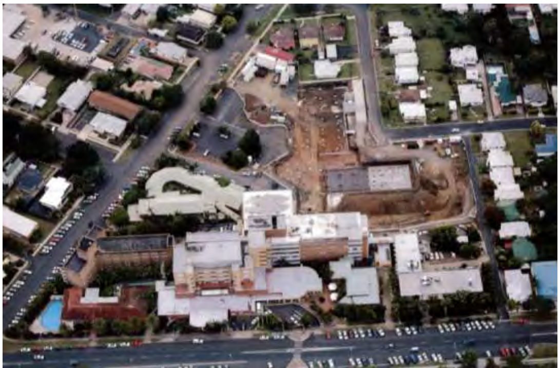
Figure 49: Excavation works as part of redevelopment planned in 1988. (Source: Courtesy of Owen Byrnes - Richmond Network Physical Resources Manager, NNSWLHD)
