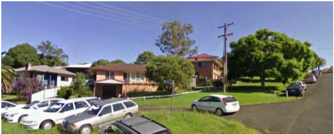
Figure 12: 28 Dalziell Street & Road Reserve
