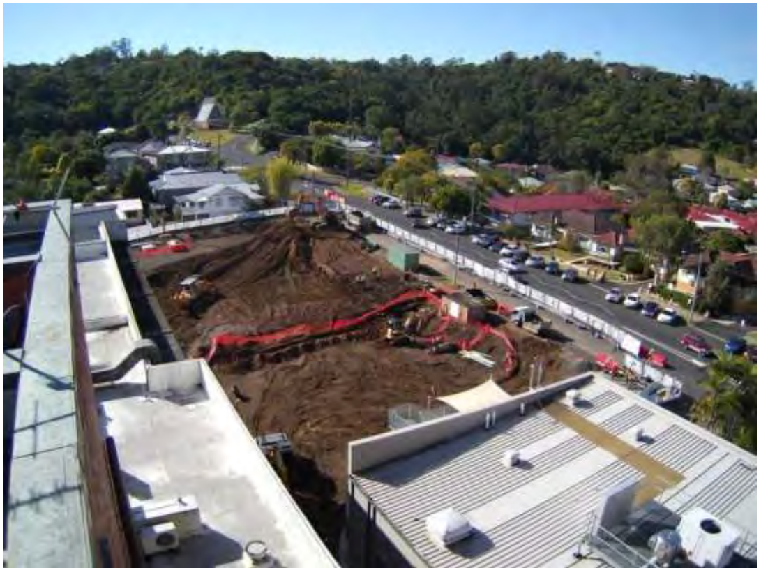
Figure 4: Excavation at LBH Site. (Source: Supplied by City Plan Strategy & Development)
