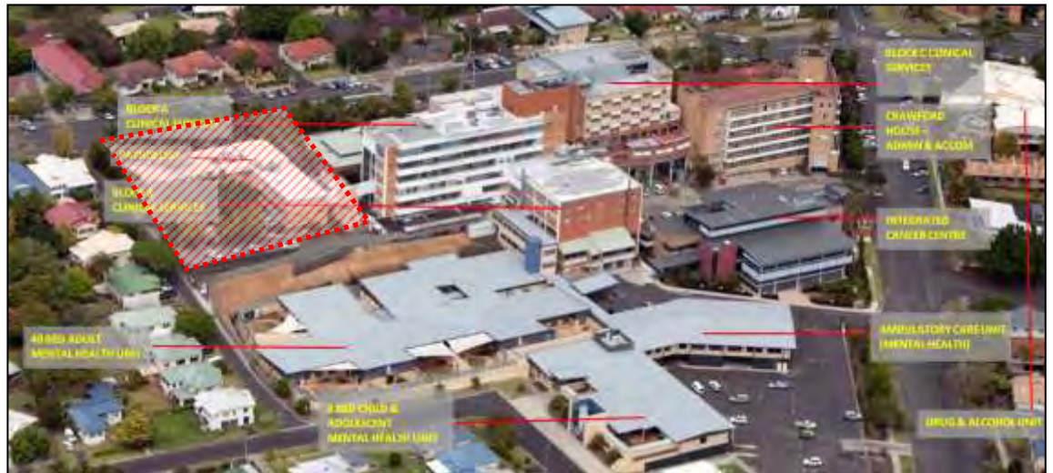
Figure 2: Lismore Base Hospital before commencement of works. The area in the red shaded area (Block P) has now been demolished as part of the Stage 3A works. (Image Source: Lismore Base Hospital Stage 3A Redevelopment Scheme Design Report Volume 1)
