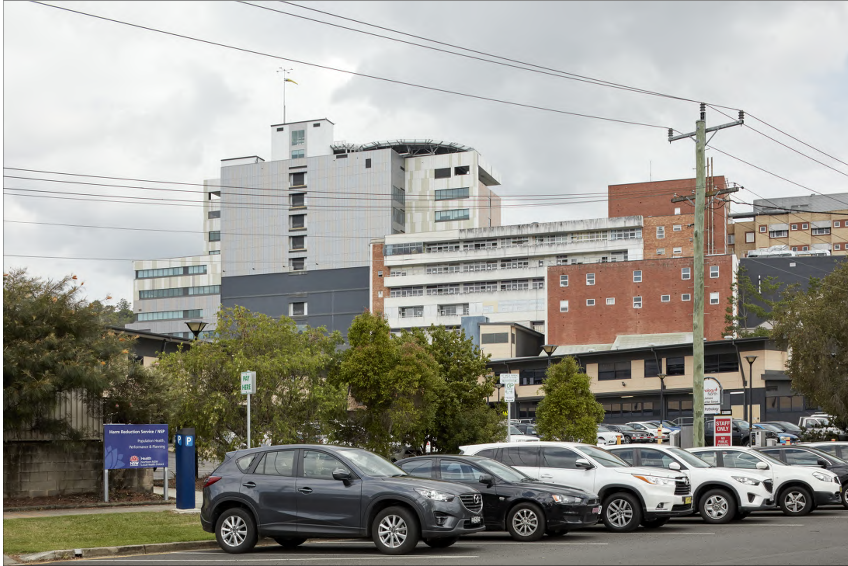
Existing - Vantage Point A
