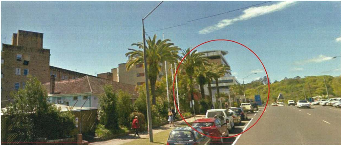
Figure 11: View of the south tower from near the corner of Hunter Street and Uralba Street (Source: Google Street View September 2016)
