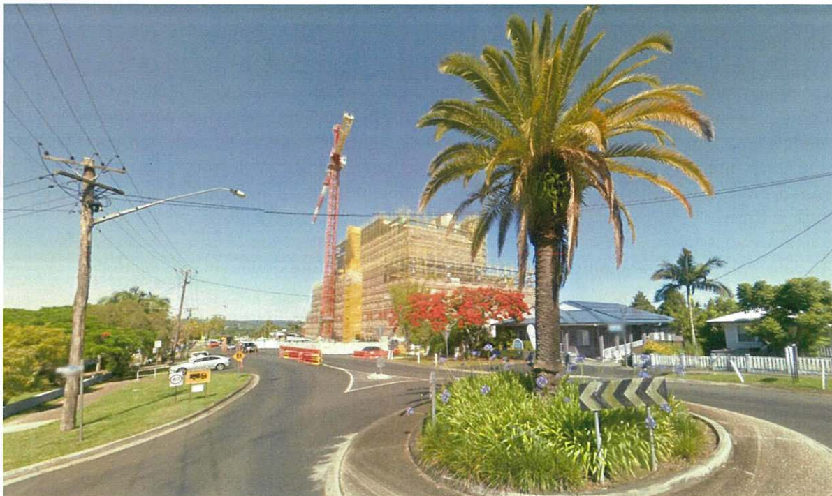
Figure 14: View of the south tower construction from Armstrong House at the south-eastern corner of Uralba Street and Dibbs Street (Source: Google Street View December 2015)
