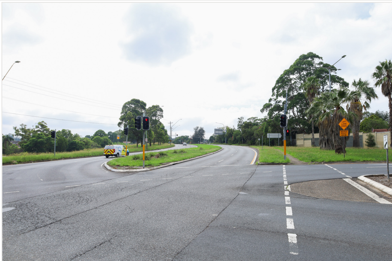
Existing site photo - Kissing Point Road
