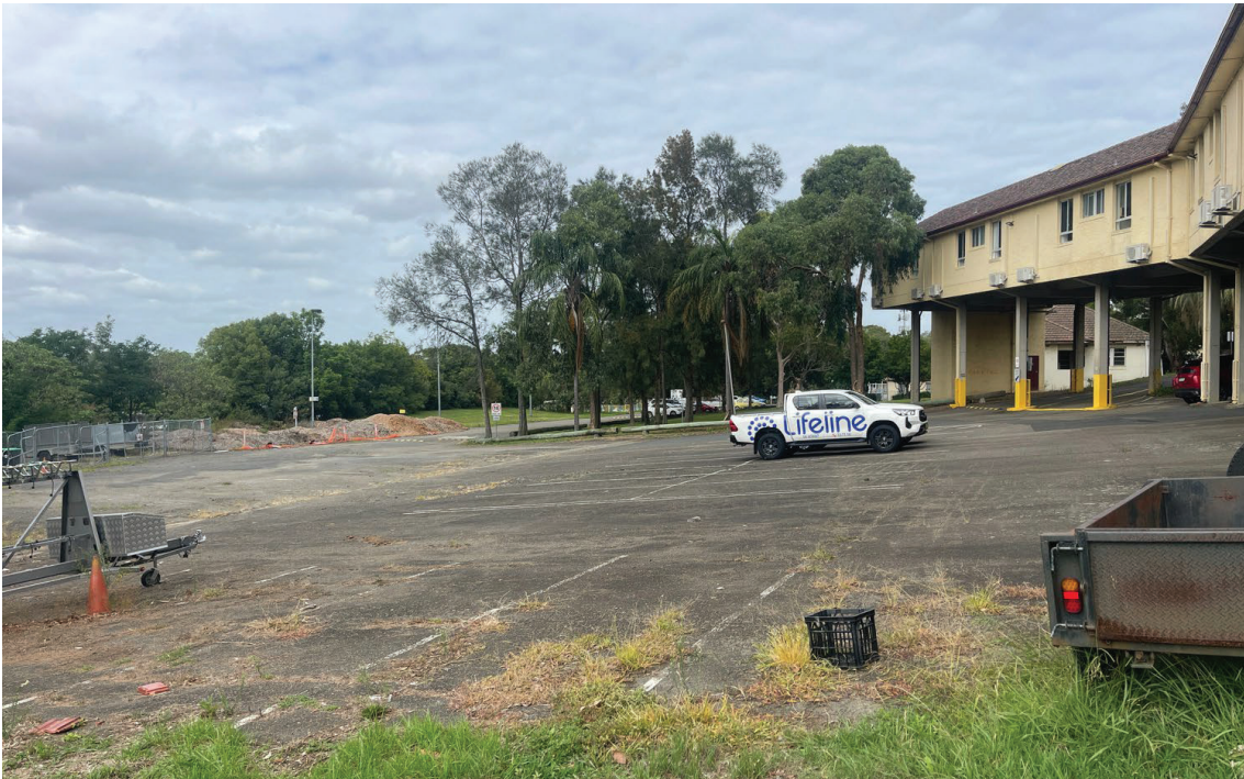
Figure 15 Tebbutt Lodge carpark extension. Imagine showing the disturbed context. Note: west facing; source: Austral.
