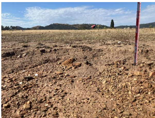
Figure 37: View north-east across a portion of BWF AS99 showing extensive sheet erosion
