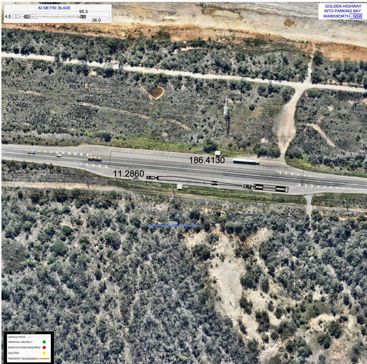
Figure 72: Warkworth parking bay
