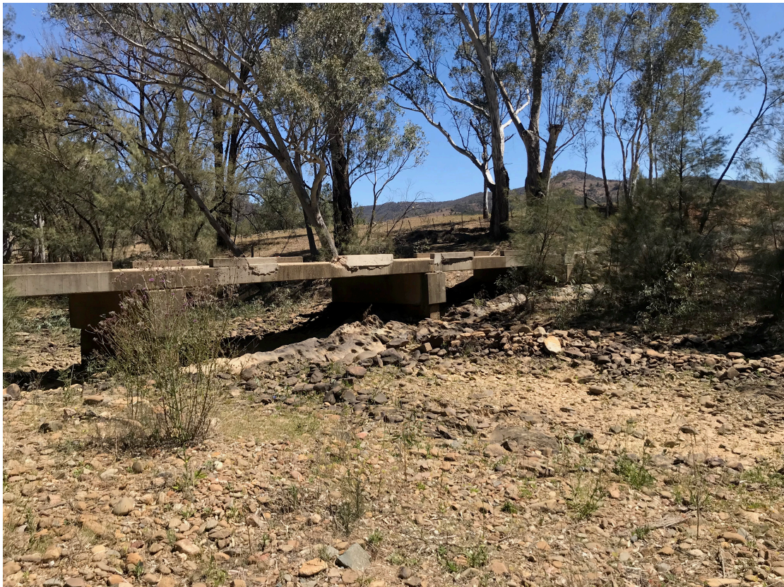
Figure 51 - Meroo River Bridge
