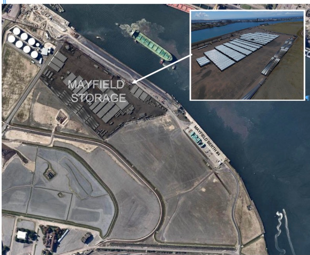
Figure 1 – Newcastle Port, Mayfield No.4 Berth
