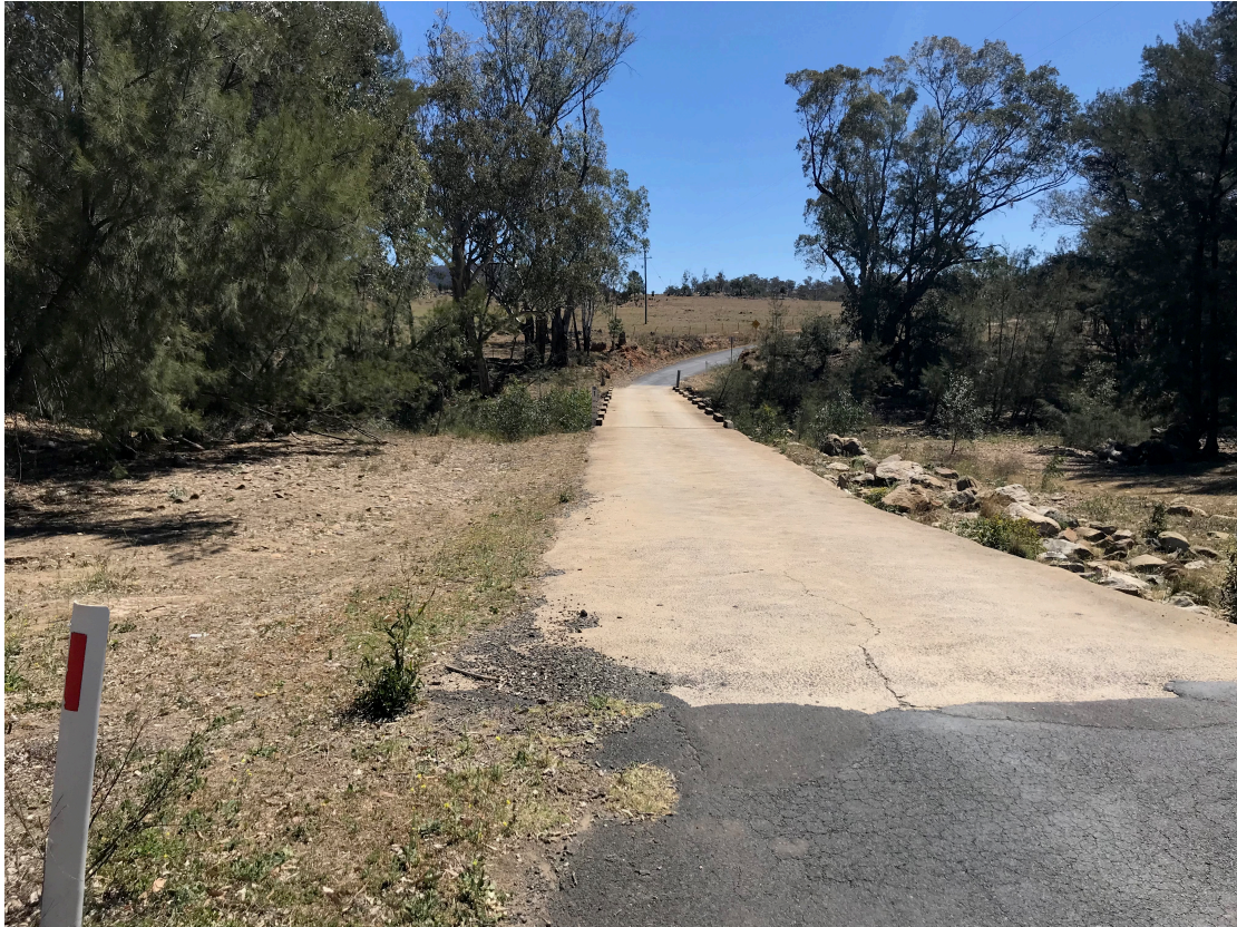
Figure 50 - Meroo River Bridge
