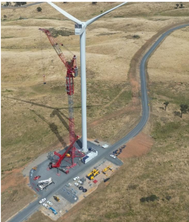
Figure 2-10: WTG Hardstand and Crane Pad
