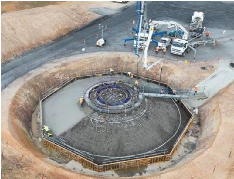
Figure 2-9: Concrete and steel reinforced WTG foundation
