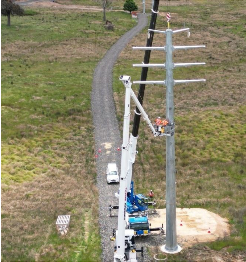
Figure 2-14: 330kV overhead powerline construction
