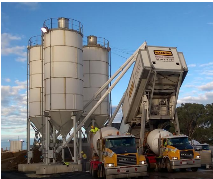
Figure 2-17: Concrete Batching Plant
