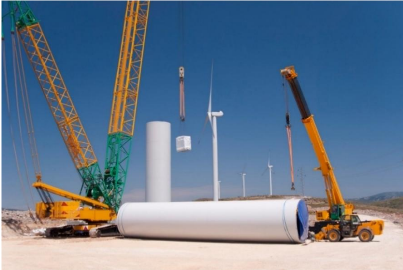
Figure 2-11: WTG tower section and installation cranes
