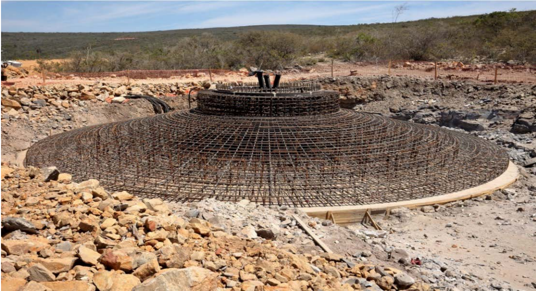
Figure 3-3: Example of gravity foundation
