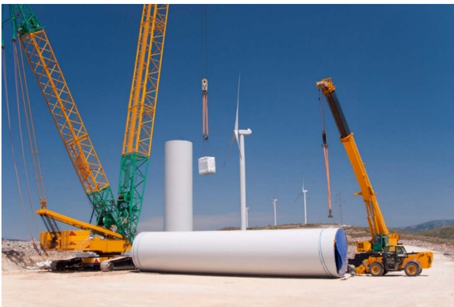
Figure 3-4: Example of WTG tower section
