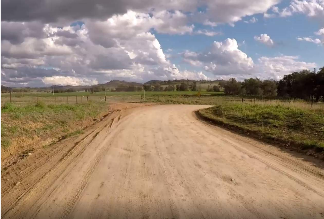
Figure 41 – Twelve Mile Rd (CH 1,000) bend
