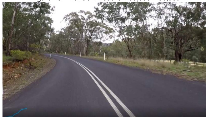
Figure 19 – Yarrabin Road CH 30,900, just after first 80 m bend.
