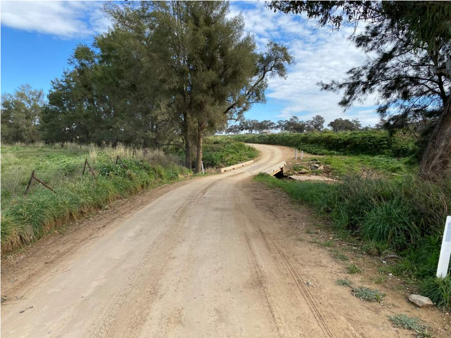
Figure 43 – Twelve Mile Rd (CH 1,150) bend
