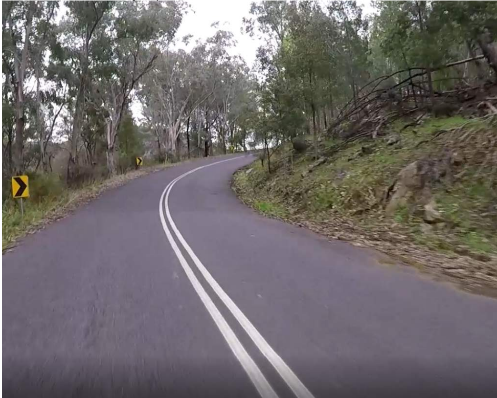
Figure 33 – Yarrabin Road CH 23,350 bend and steep crest
