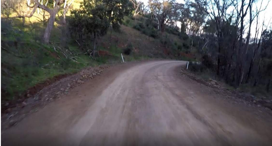
Figure 69 – Yarrabin Rd (CH 14,200), s-bend with drop off on right
