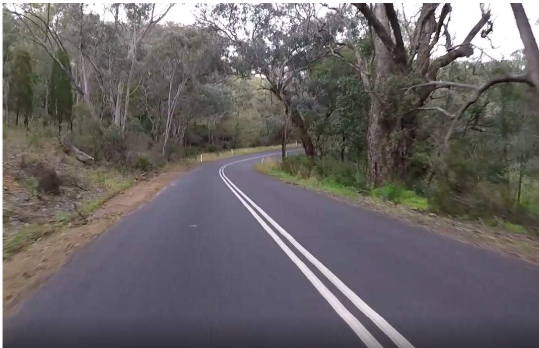
Figure 15 – Yarrabin Road CH 31,650 tight bend and dense vegetation
