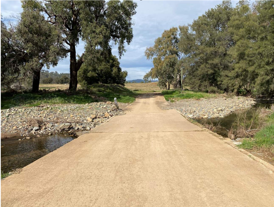
Figure 71 – Yarrabin Rd (CH 16,500), concrete floodway
