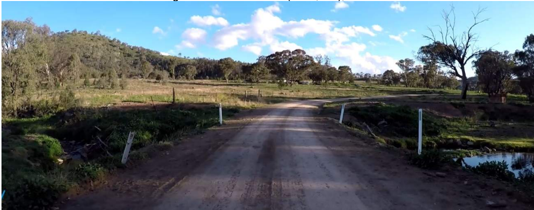
Figure 57 – Yarrabin Rd (CH 4,550), culvert
