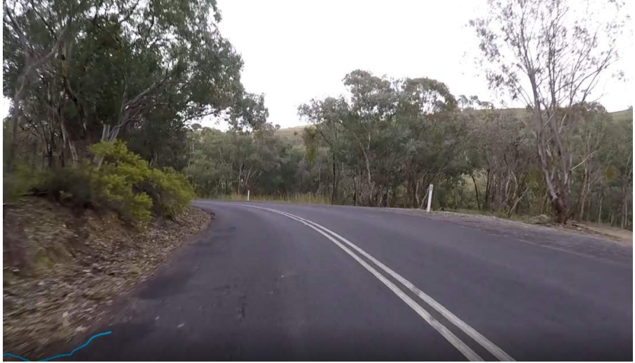
Figure 22 – Yarrabin Road CH 29,650
