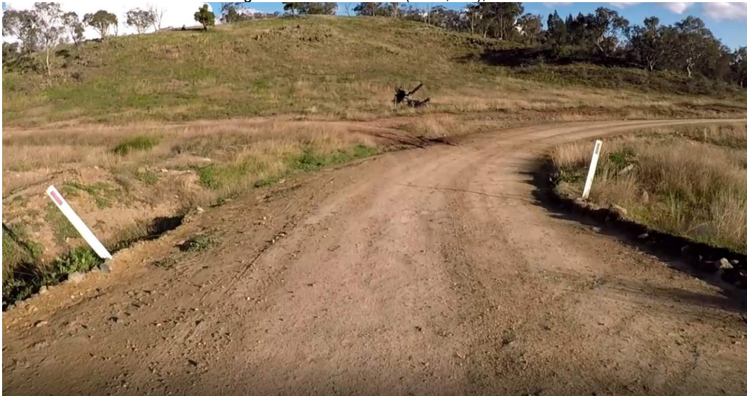
Figure 55 – Yarrabin Rd (CH 3,750), bend and culvert crossing
