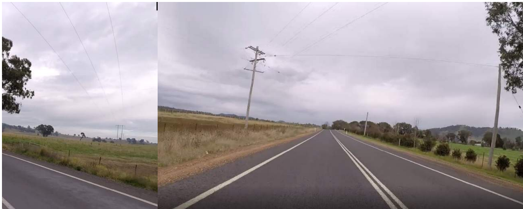
Figure 35 – Example Hill End Road overhead line crossings. Left : CH 1,300. Right : CH 6,400.
