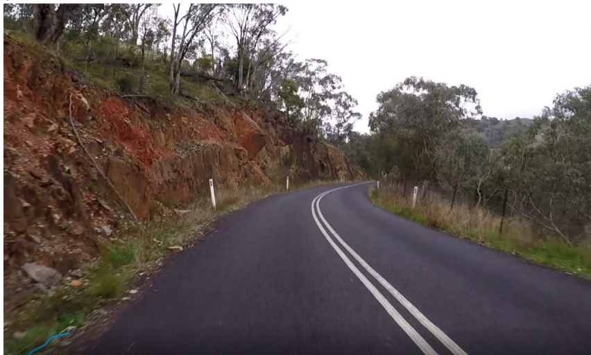
Figure 20 – Yarrabin Road CH 30,750. Rock wall and sharp drop off.
