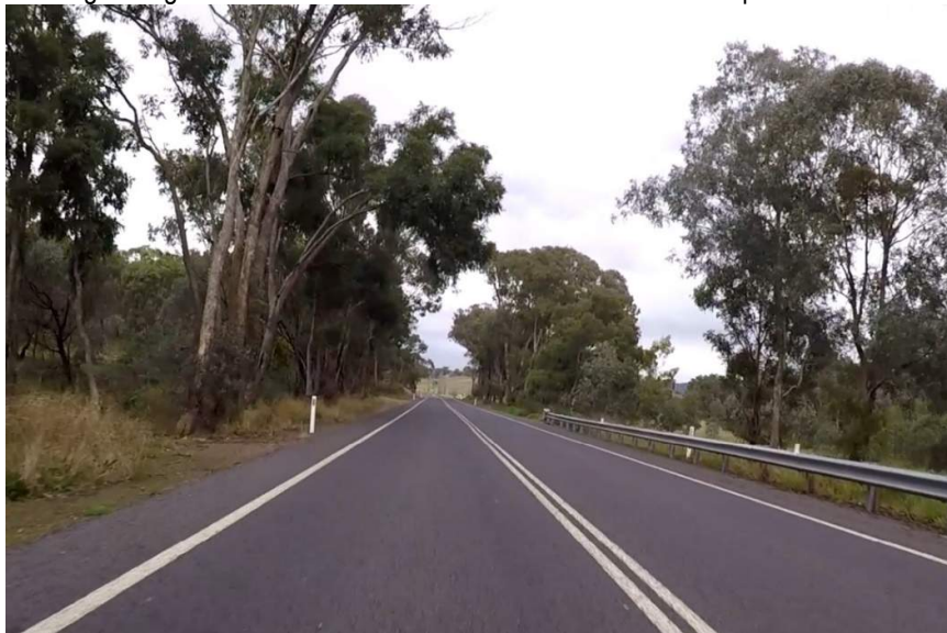
Figure 3 – Example of tree overhang which may require trimming (Hill End Rd, approx. CH9300)
