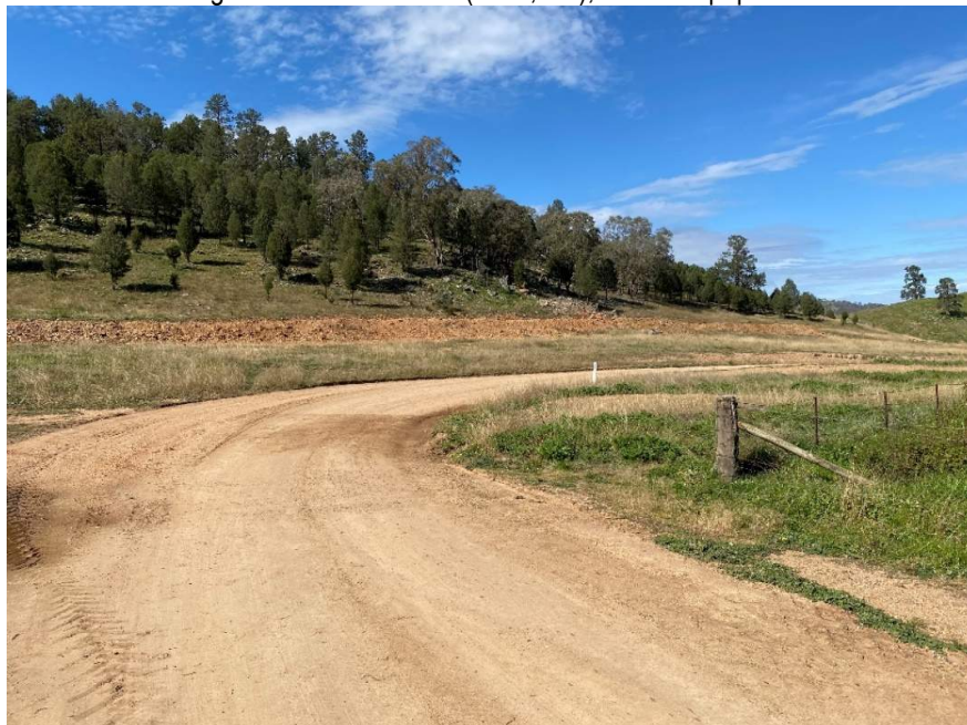
Figure 49 – Yarrabin Rd (CH 1,000), bend and fence
