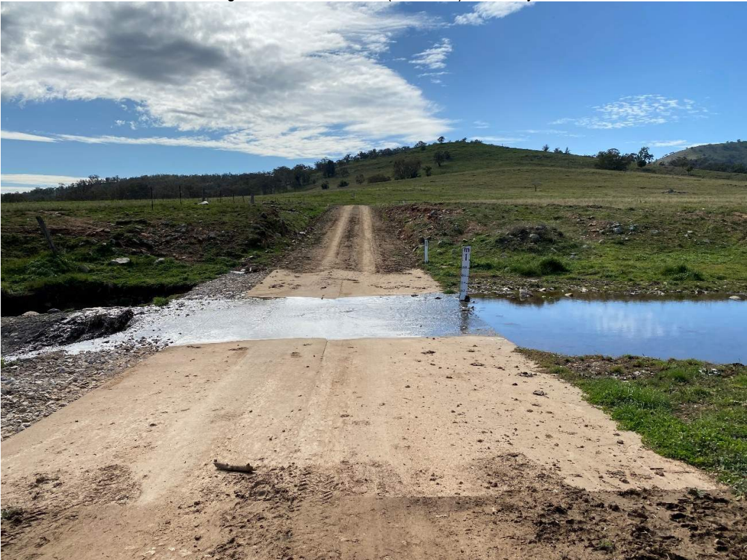
Figure 64 – Yarrabin Rd (CH 7,925), floodway and vertical curve
