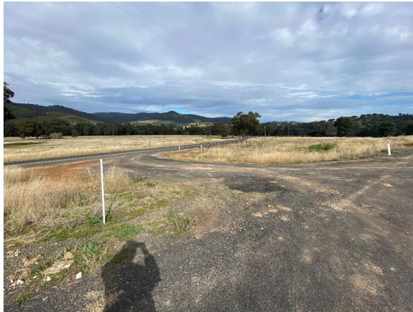
Figure 76 – Yarrabin Rd & Burrendong Dam Rd intersection
