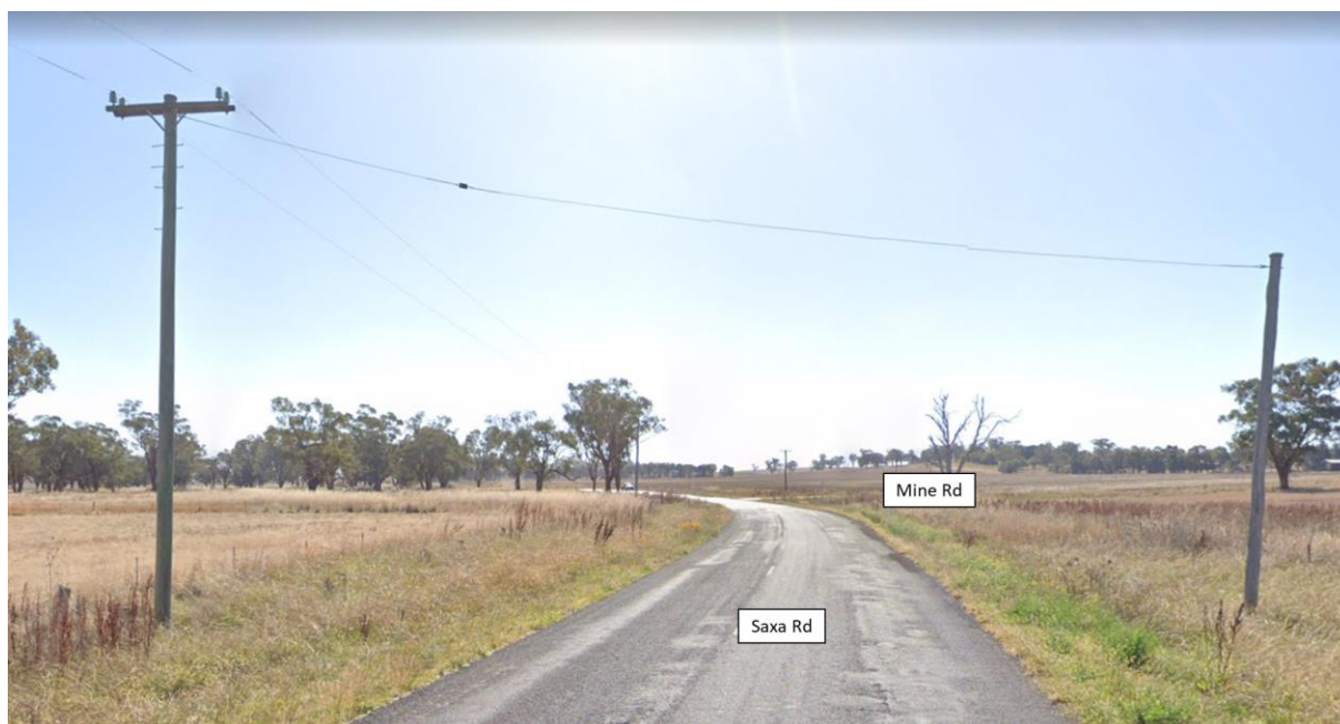
Figure 3.6 – Intersection of Saxa Road and Mine Road, Maryvale
