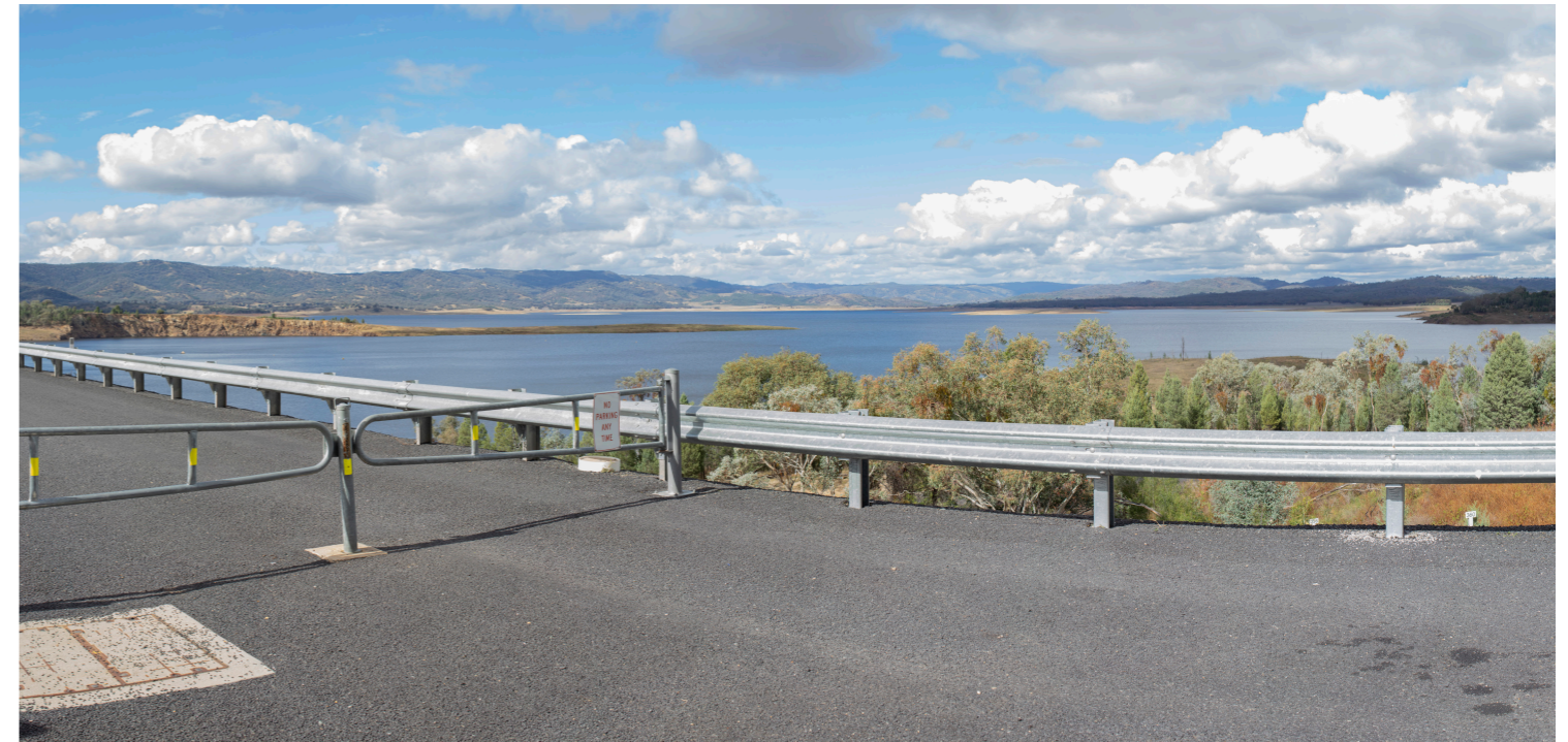
Image B7. View across Lake Burrendong from the Burrendong Dam Wall
