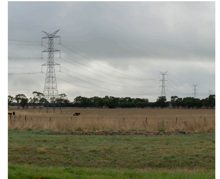
Image 2 Typical Transmission Line
