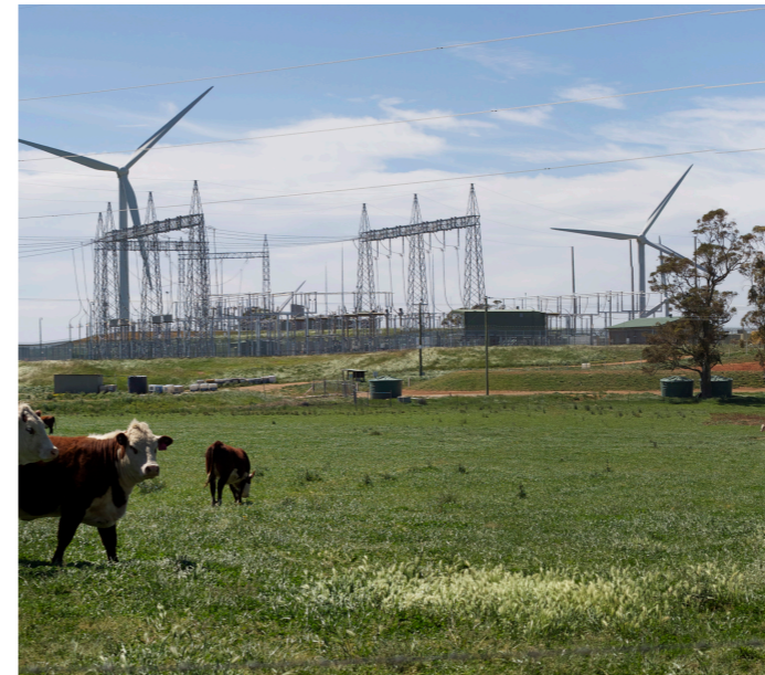
Image 1 Typical Substation (Gullen Range Wind Farm)
