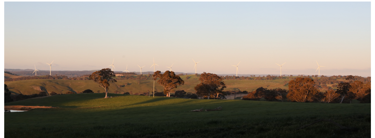
Image 15. Photo of Gullen Range Wind Farm at dusk, looking in a east direction with sun on WTGs
