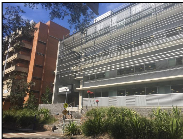
Photo 3 – Medical Sciences located north of the building site (looking southeast)
