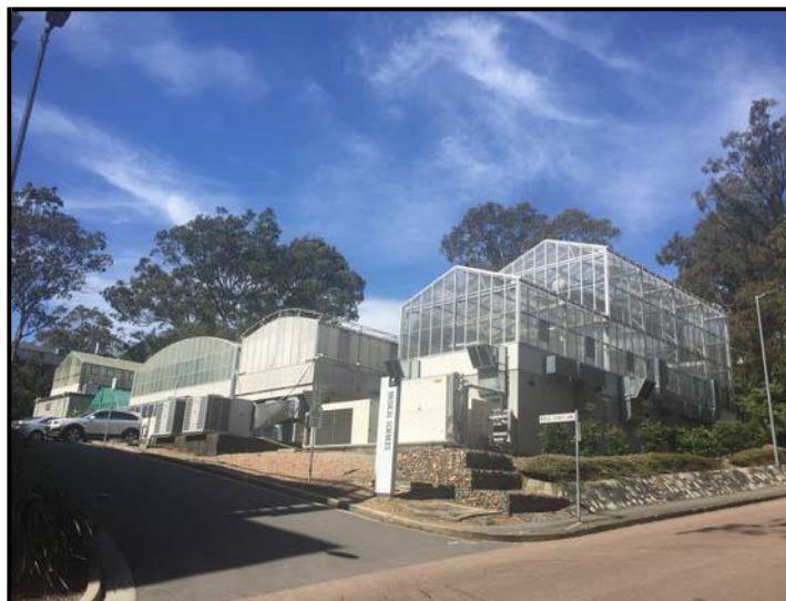
Photo 1 – Existing Glass Houses (looking southeast)
