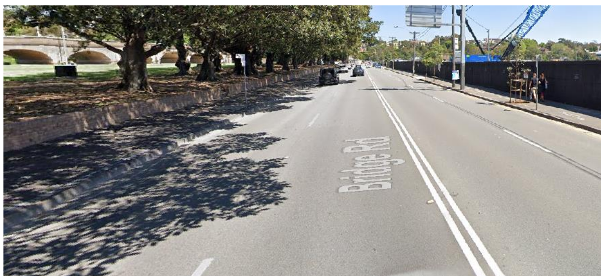
Figure 6: Street view of the Existing Road Network – Bridge Road (Westbound)
