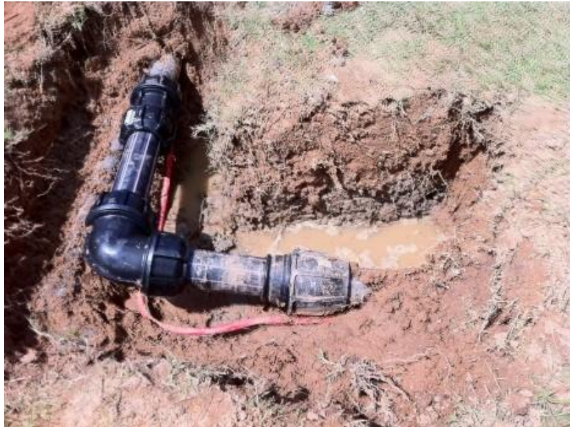
Image 2 – Mainline installed too shallow and damaged by mower
