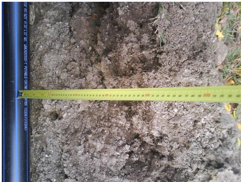
Image 3 – Mainlines to be installed at minimum 450mm below surface
