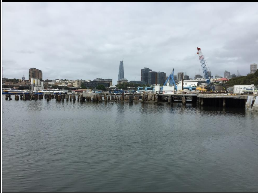
PHOTOGRAPH 2: THE INVESTIGATION AREA – FACING NORTH-EAST
