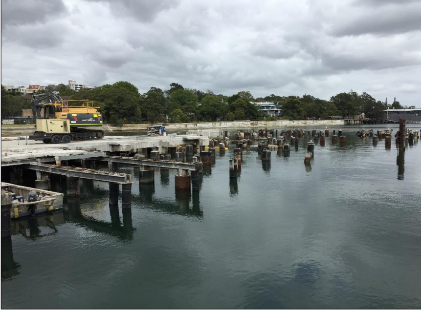
PHOTOGRAPH 1: THE INVESTIGATION AREA – FACING NORTH-WEST
