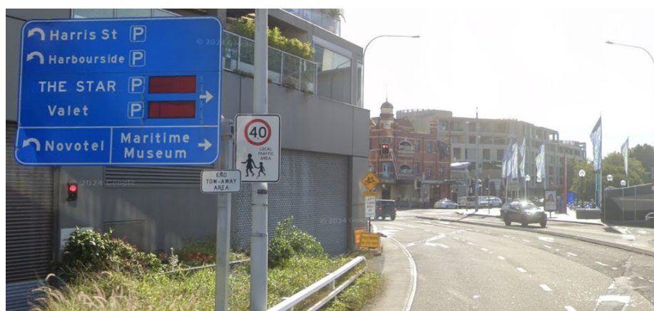
Figure 13 - Existing parking signage on Darling Drive
