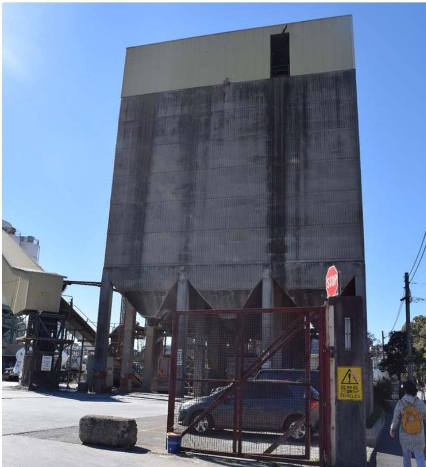
Figure 24: The western façade of the concrete cube like silo structure.
