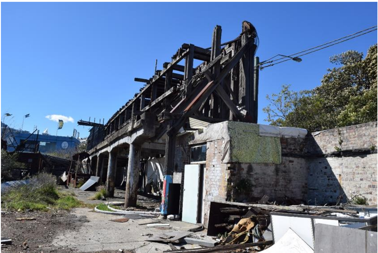
Figure 12: The western end of the former coal loader.
