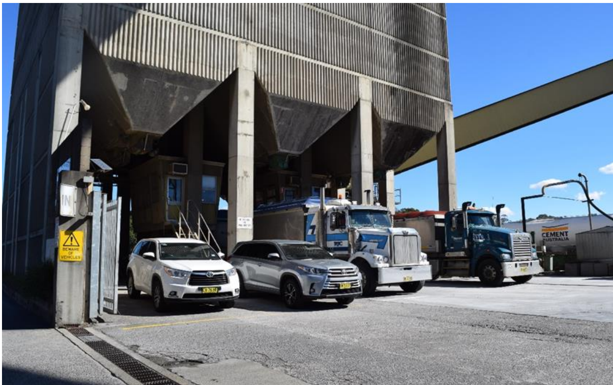
Figure 22: The Hanson Heidelberg cement manufacturing plant as viewed from the south eastern Bridge Road entrance. This view is looking north west towards the base of the large cube like concrete structure.
