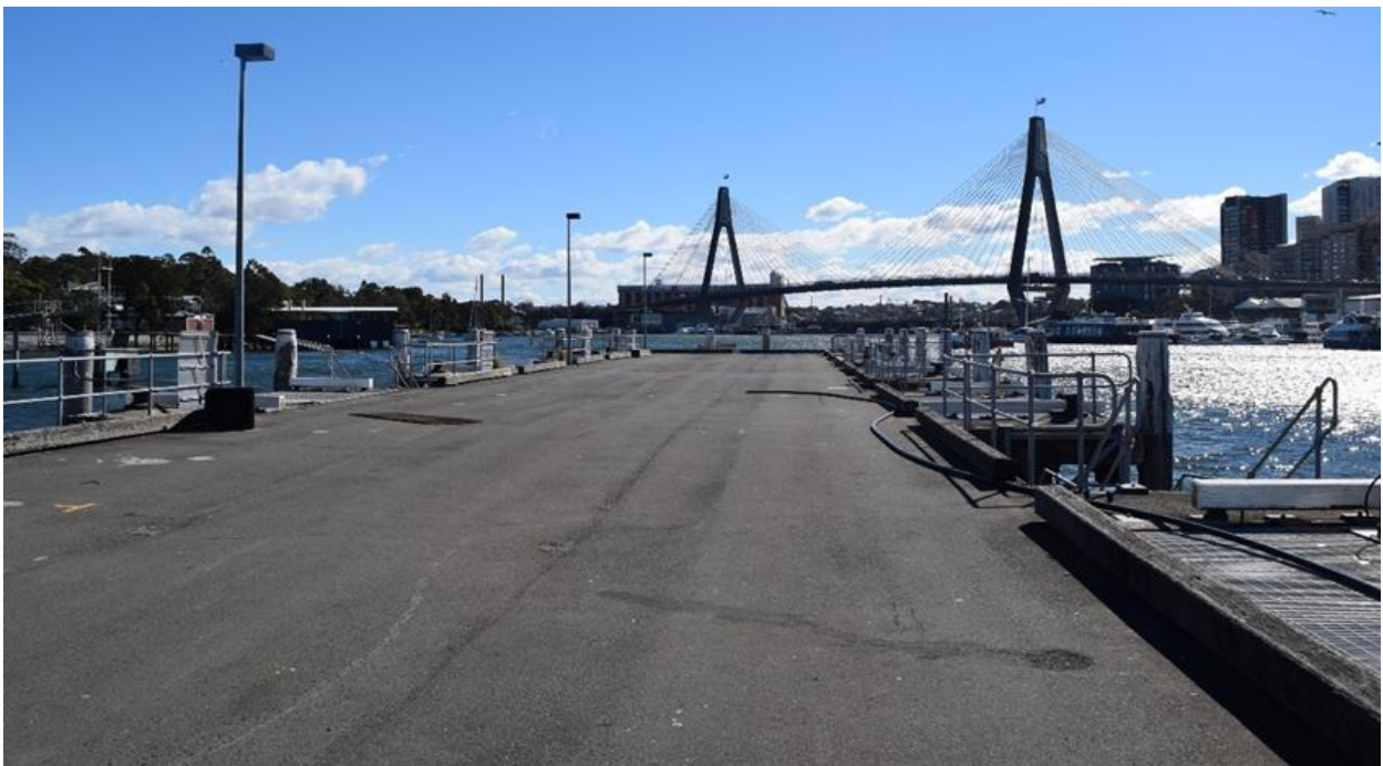
Figure 19: Looking north along the concrete wharf located within B2
