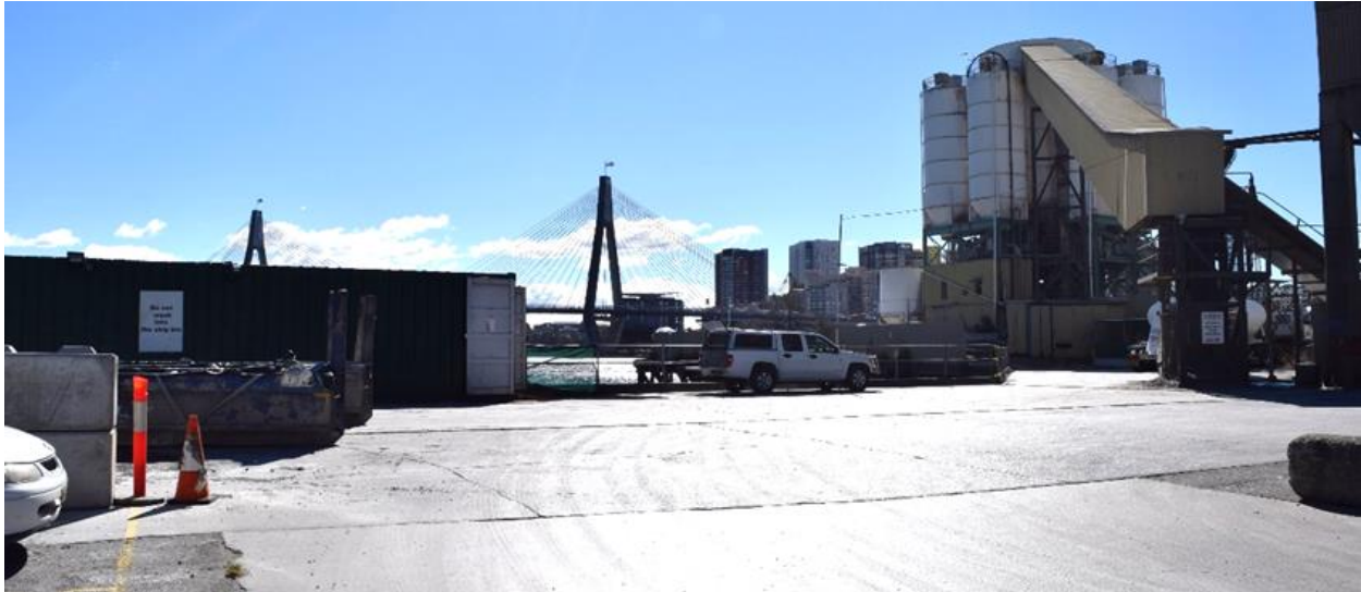
Figure 23: The south western entrance to B2, looking north. Note Pymont Bridge is visible in the background.
