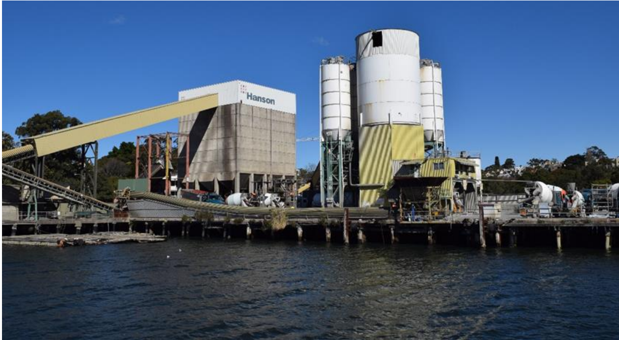
Figure 21: The eastern extent of Berth no. B3, as viewed from within Berth B2.
