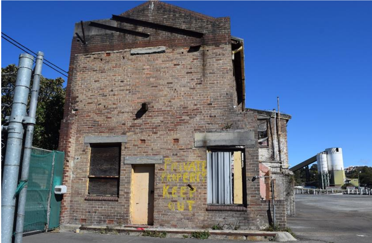
Figure 16: The eastern façade of the former office/ weighbridge building.
