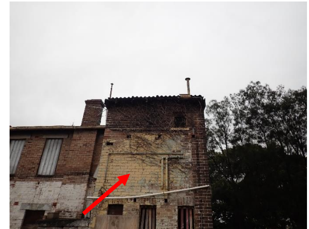
Photo 27: Lot 4, Old Office Building, lead based cream paint to the external north wall
