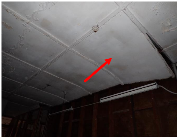
Photo 28: Lot 4, Old Office Building, lead based white paint to the ground floor ceiling
