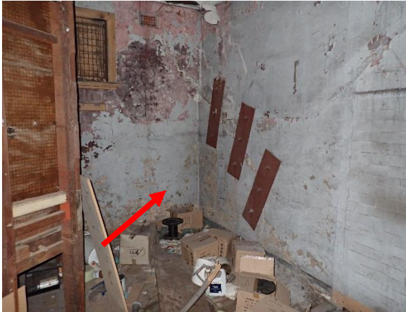
Photo 31: Lot 4, Old Office Building, lead based white paint to the ground floor internal brick walls
