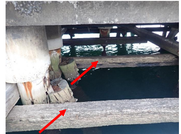
Photo 12: Lot 4, lead based white paint to the timber beams of the pier
