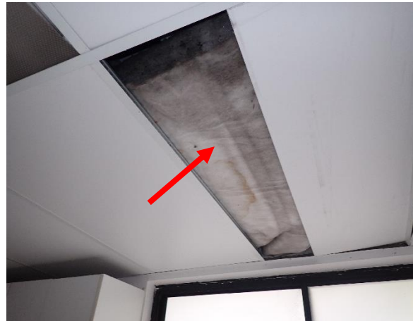
Photo 41: Lot 4, Site Office, assumed SMF insulation throughout the roof void
