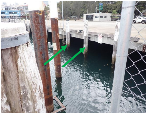
Photo 52: Lot 4 wharf, no timber treatments were identified to the timber piles
