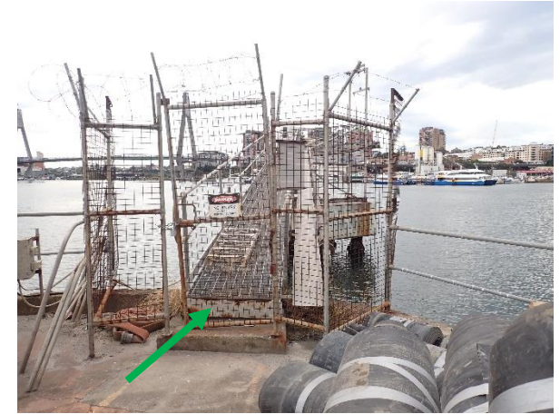
Photo 45: Lot 5, non-lead based white paint to the pier extending from the northern portion of the lot
