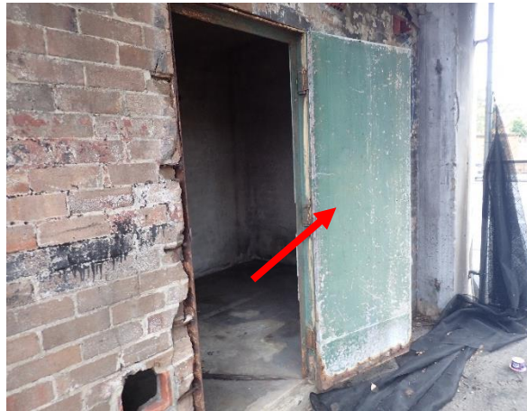
Photo 5: Lot 3, lead based green paint to the store room door
