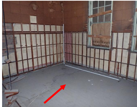
Photo 26: Lot 4, Old Office Building, lead containing dust throughout the first floor
