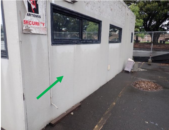
Photo 37: Lot 4, Site Office, non-asbestos containing fibre cement sheeting to the external walls
