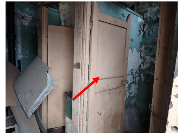
Photo 30: Lot 4, Old Office Building, lead based yellow/orange paint to the ground floor toilet timber doors and frames
