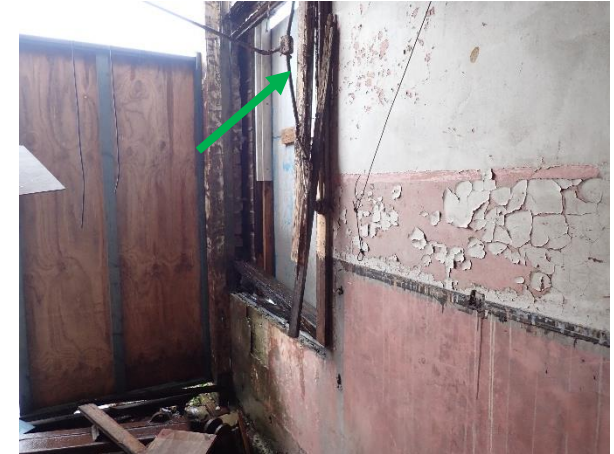
Photo 21: Lot 4, Old Office Building, non-asbestos containing red and black cable sheath to redundant electrical wiring
