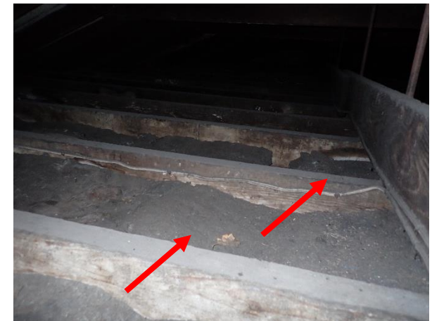
Photo 24: Lot 4, Old Office Building, lead containing dust and SMF insulation throughout the roof void
