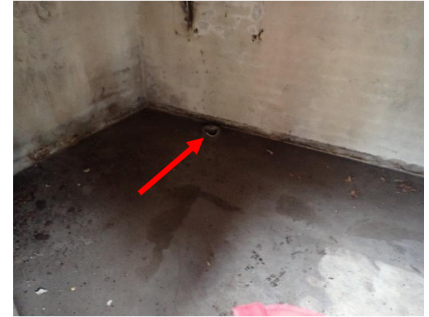
Photo 3: Lot 3, asbestos containing fibre cement conduit penetrating the floor of the store room
