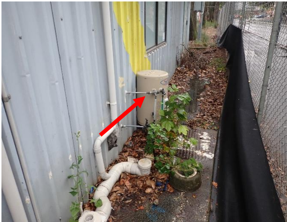
Photo 40: Lot 4, Site Office, assumed SMF insulation to the hot water system
