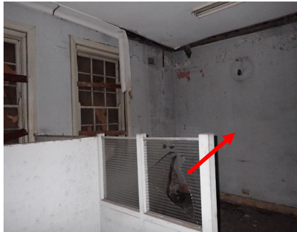
Photo 35: Lot 4, Old Office Building, lead based blue paint to the first floor main room walls
