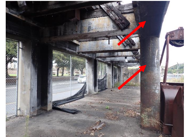
Photo 6: Lot 3, lead based black paint to the columns and beams of the timber structure
