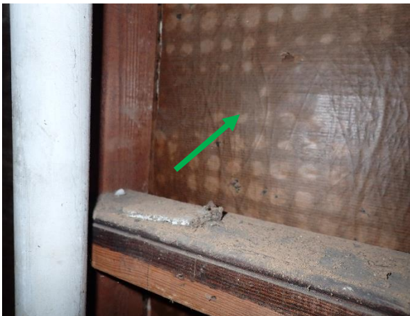
Photo 22: Lot 4, Old Office Building, non-asbestos containing bituminous backing to the cement rendered walls of the stairwell
