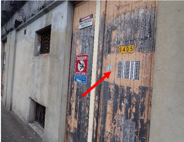
Photo 7: Lot 3, lead based yellow paint to the substation timber doors
