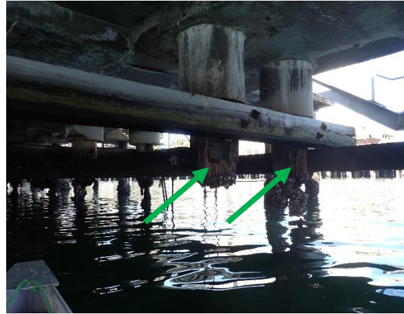
Photo 50: Lot 4 pier, no timber treatments were identified to the timber piles
