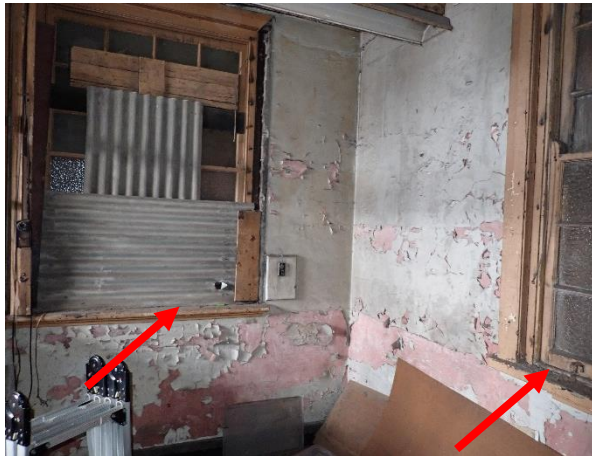
Photo 25: Lot 4, Old Office Building, lead containing dust to the ground floor window sills
