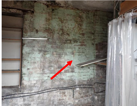
Photo 8: Lot 3, lead based blue paint to the shower room walls
