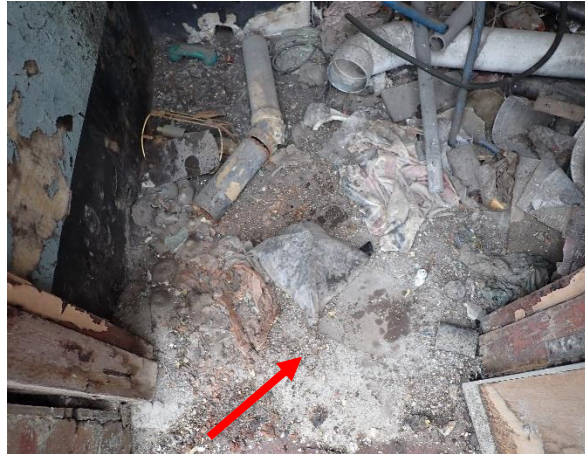
Photo 20: Lot 4, Old Office Building, asbestos containing and lead containing settled dust to the floor of the ground floor toilets
