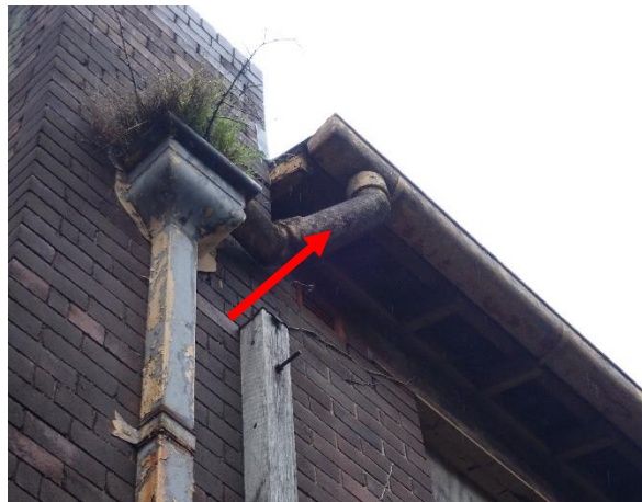
Photo 17: Lot 4, Old Office Building, assumed asbestos containing fibre cement downpipe
