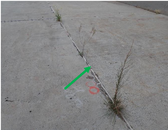
Photo 10: Lot 4, non-asbestos containing mastic to the concrete expansion joint
