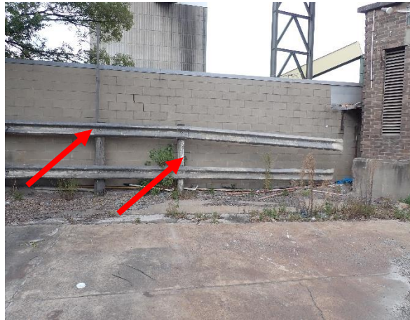
Photo 11: Lot 4, lead based white paint to the metal and timber barrier at the SW end of the lot
