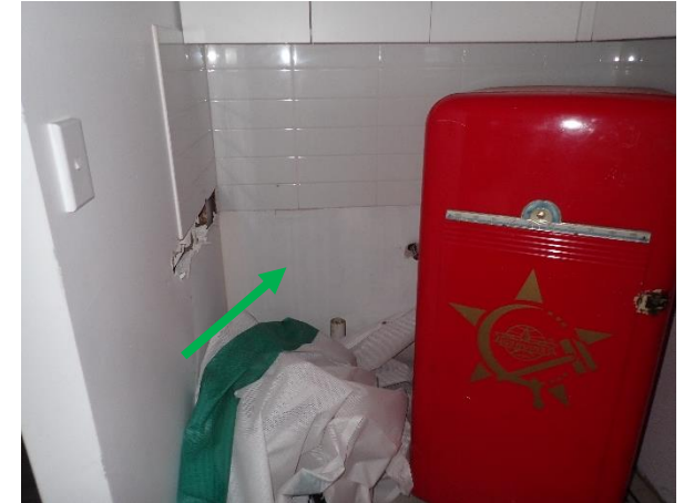
Photo 39: Lot 4, Site Office, non-asbestos containing fibre cement sheeting to the former kitchenette
