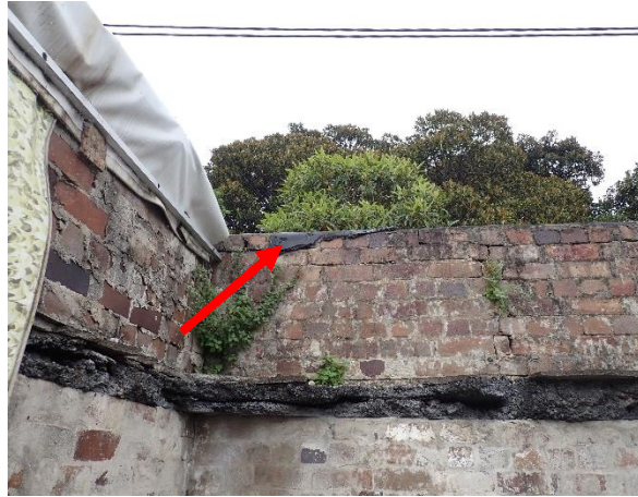
Photo 2: Lot 3, asbestos containing bituminous membrane on top of the brick wall adjacent the shower room
