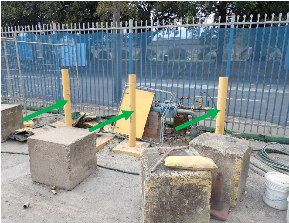
Photo 46: Lot 5, non-lead based yellow paint to the bollards in the southern portion
