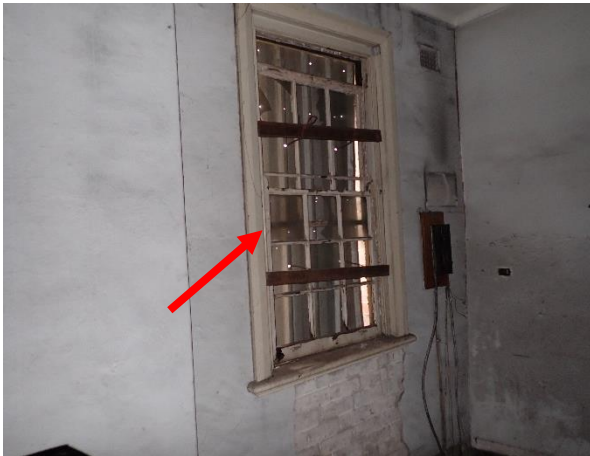
Photo 34: Lot 4, Old Office Building, lead based white paint to the first floor main room windows
