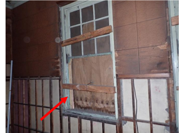
Photo 33: Lot 4, Old Office Building, lead based green paint for the first floor east room windows
