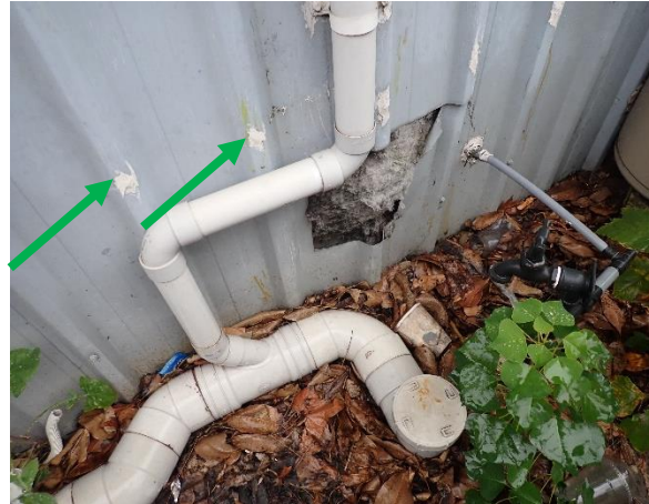
Photo 38: Lot 4, Site Office, non-asbestos containing mastic to the external metal walls
