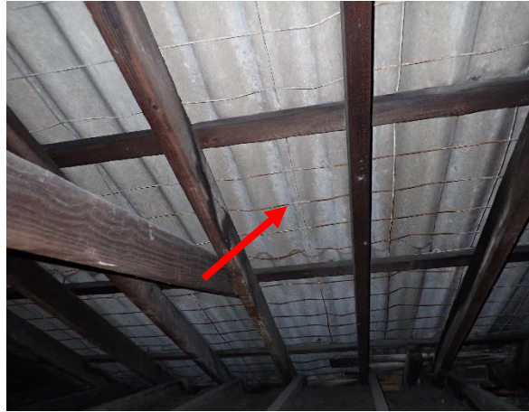
Photo 14: Lot 4, Old Office Building, asbestos containing corrugated fibre cement roof (internal surface)
