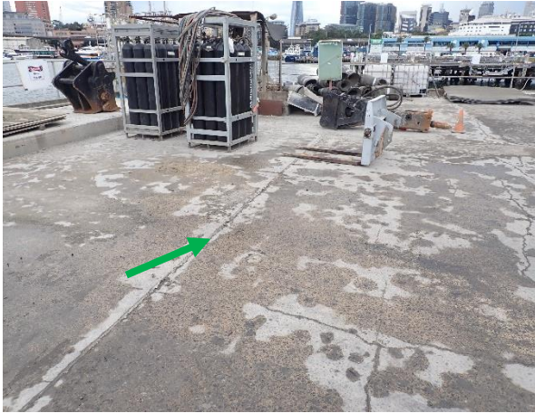
Photo 43: Lot 5, non-asbestos containing mastic to the expansion joint in the northern portion
