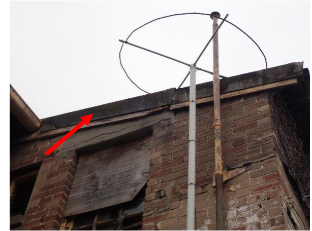
Photo 15: Lot 4, Old Office Building, asbestos containing fibre cement roof barge capping
