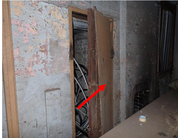
Photo 32: Lot 4, Old Office Building, lead based brown paint to the north store room door
