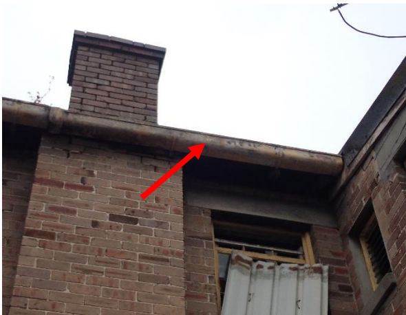
Photo 16: Lot 4, Old Office Building, assumed asbestos containing fibre cement gutters
