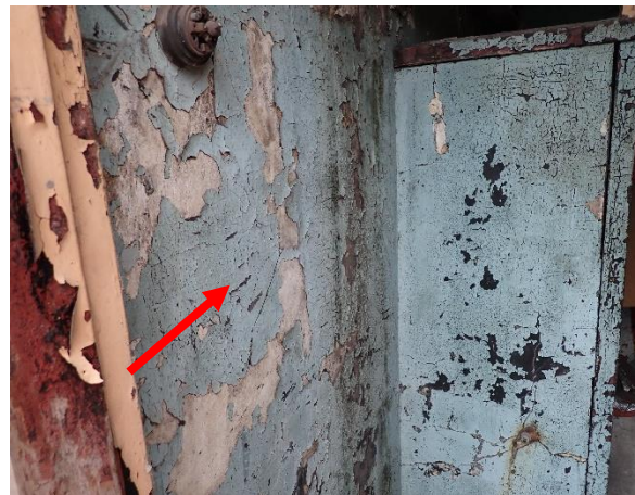
Photo 29: Lot 4, Old Office Building, lead based blue paint to the ground floor toilet walls
