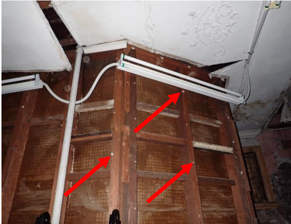
Photo 19: Lot 4, Old Office Building, asbestos containing fibre cement fragments to the timber studs and behind nails on the south wall of the main room (ground floor)
