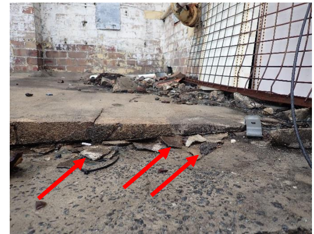
Photo 18: Lot 4, Old Office Building, asbestos containing mixed fibre cement debris on top of the concrete roof to the north store room
