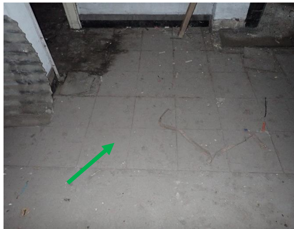
Photo 23: Lot 4, Old Office Building, non-asbestos containing black vinyl tiles and paper backing to the floor covering on the first floor
