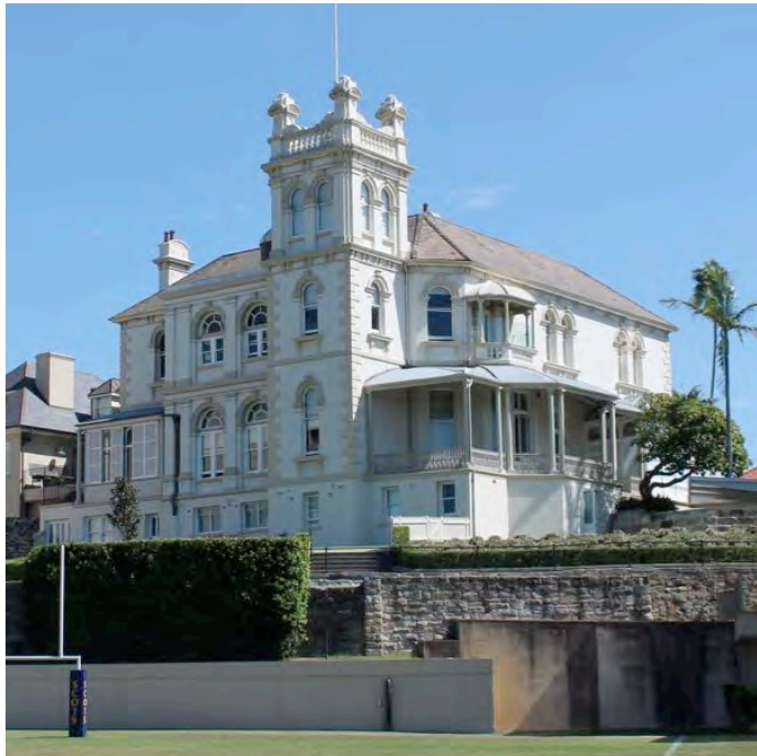
Figure 8.1 Aspinall House looking southwest from the Oval
