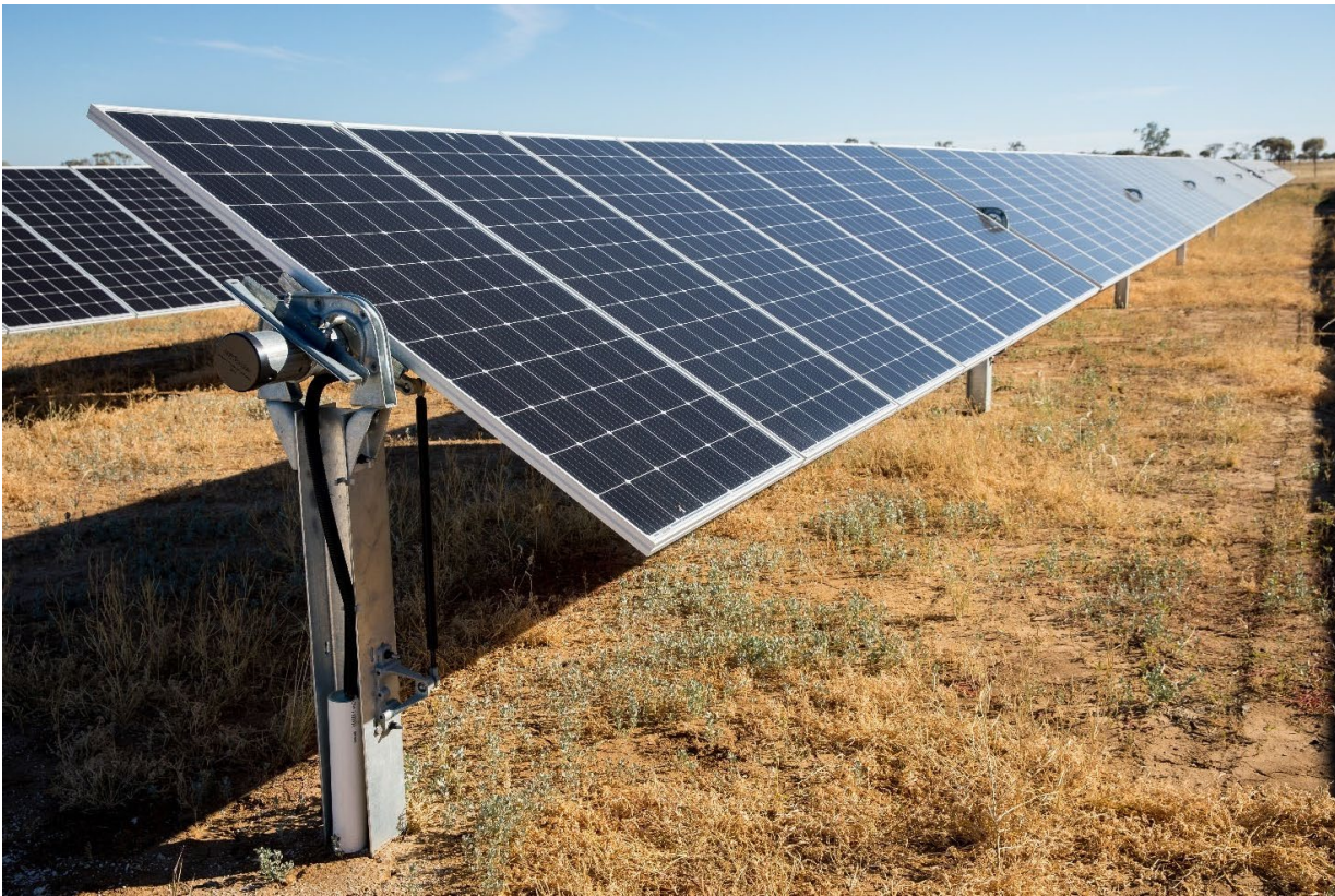
Photograph 2.1 PV panel row with single axis tracker
