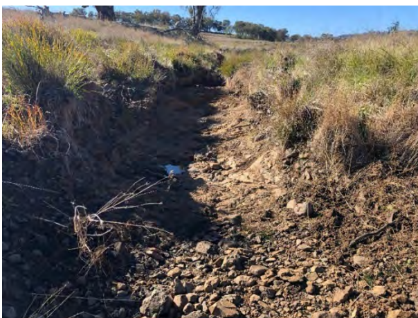
Plate 8.7 Rocky base, Jessie Creek. TR16, view south
