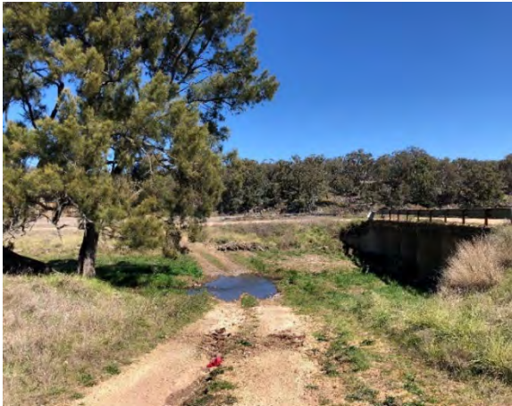
Plate 8.15 Swan Brook, bridge crossing, view south
