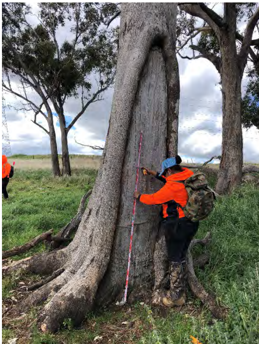
Plate 8.43 SSF-ST9: Elongated scar that extends to the ground
