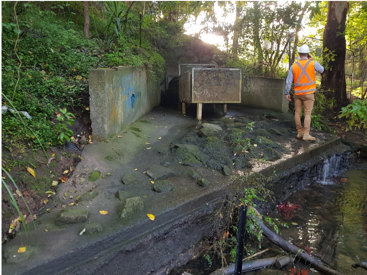
Figure 3: Existing 1200mm Headwall
