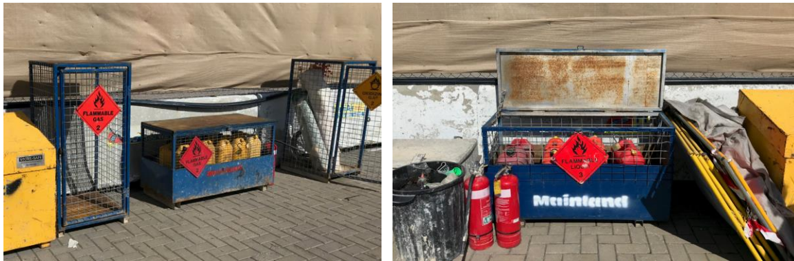
Figure 4.7.6.1.2– Spare Fuel Contained in Bunded Flammable Cages
