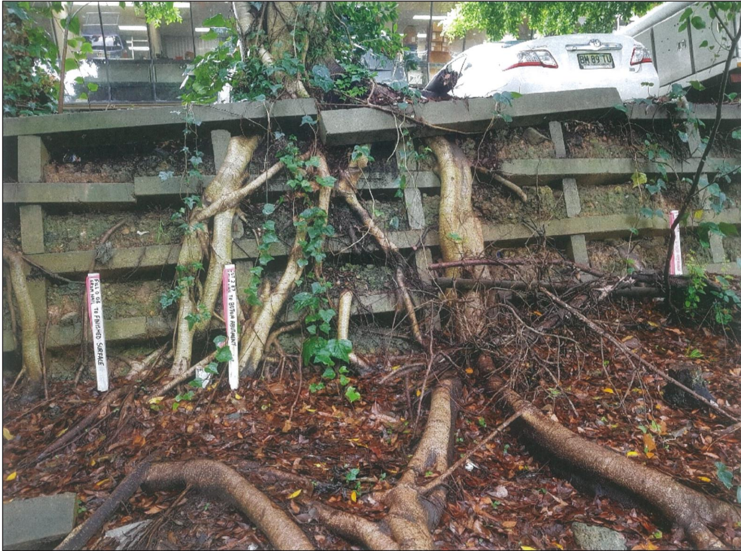
Figure 3: Large roots traversing down crib wall (photo provided by Christie Civil on 3 March 2022)
