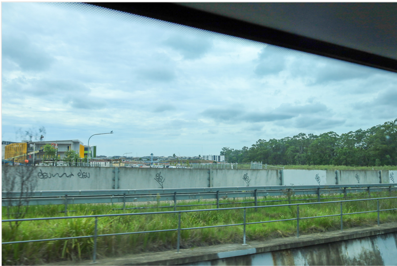
Existing site photo - Oxley Street
