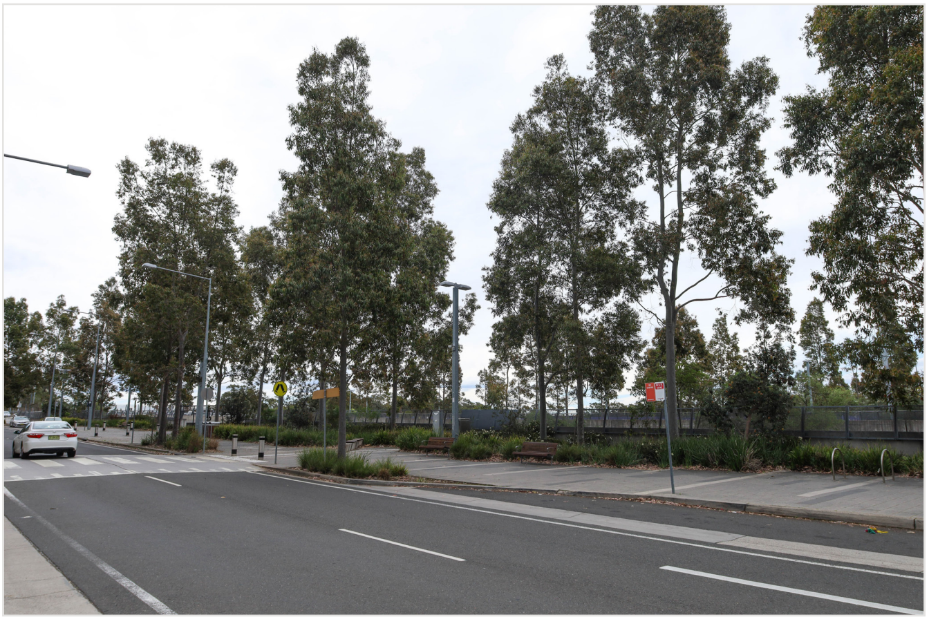
Existing site photo - Edmondson Park South
