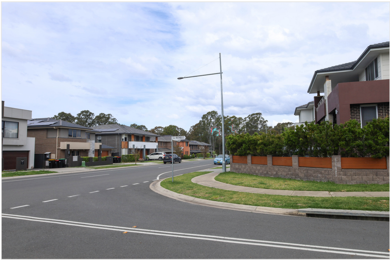
Visual impact in cyan with red outline, Concept Plan Mod 5 in blue outline
