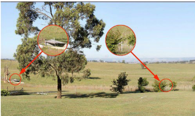
Physical 3000mm site poles placed at lot corners
