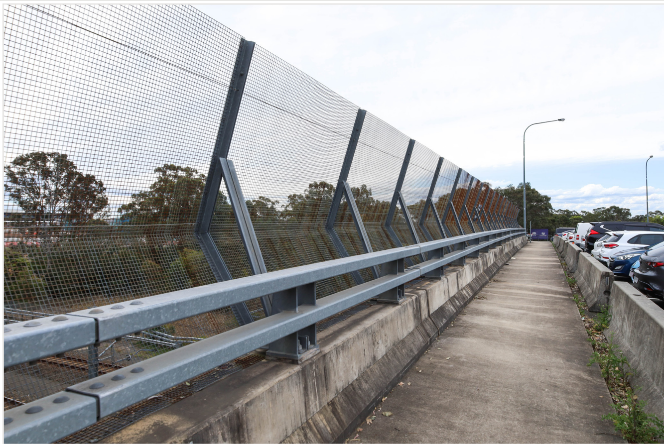
Existing site photo - Edmondson Park
