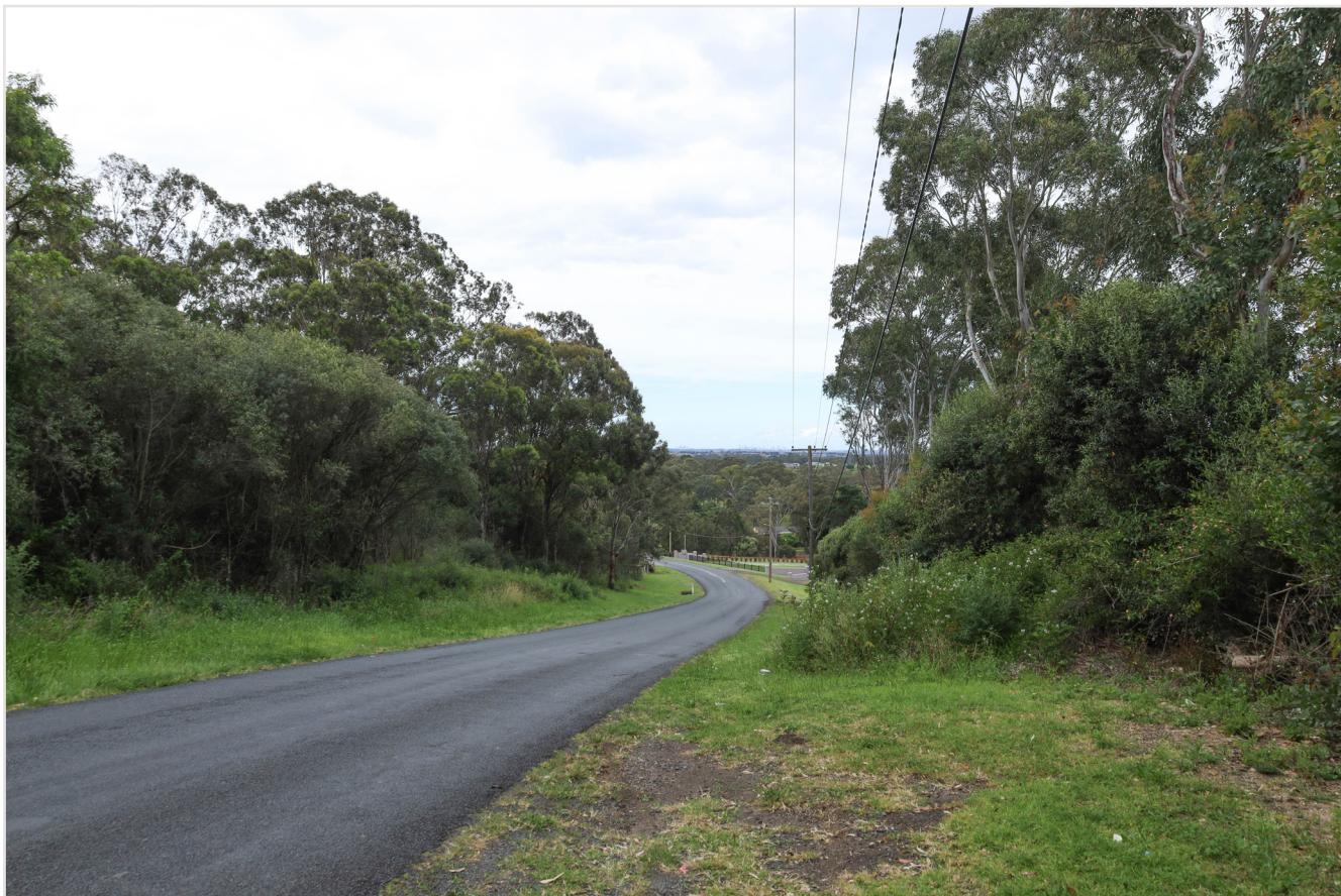
Existing site photo - Springmead Drive
