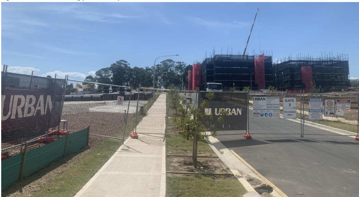
Figure 20: Gate delineating private and public road access
