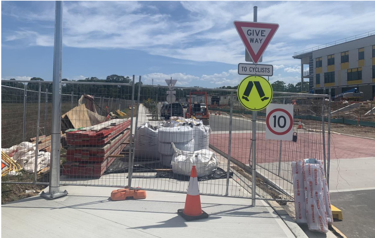
Figure 19: Horrie Rd footpath intersection with Buchan Ave
