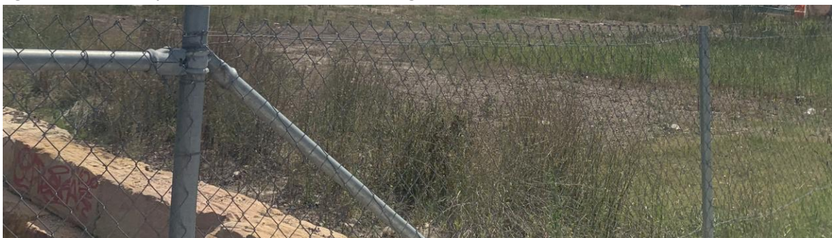
Figure 24: Graffiti and pieces of rubbish within the site along Buchan Ave
