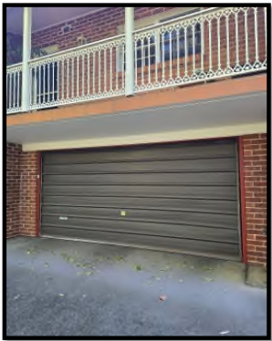
View of: Garage with brick walls and metal gates observed under each unit.
