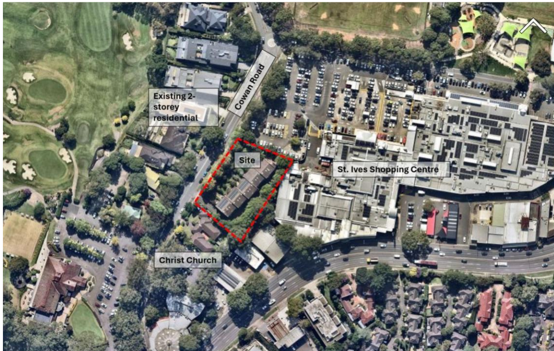
Figure 1 – Site Location (Source: Nearmap 2025)
