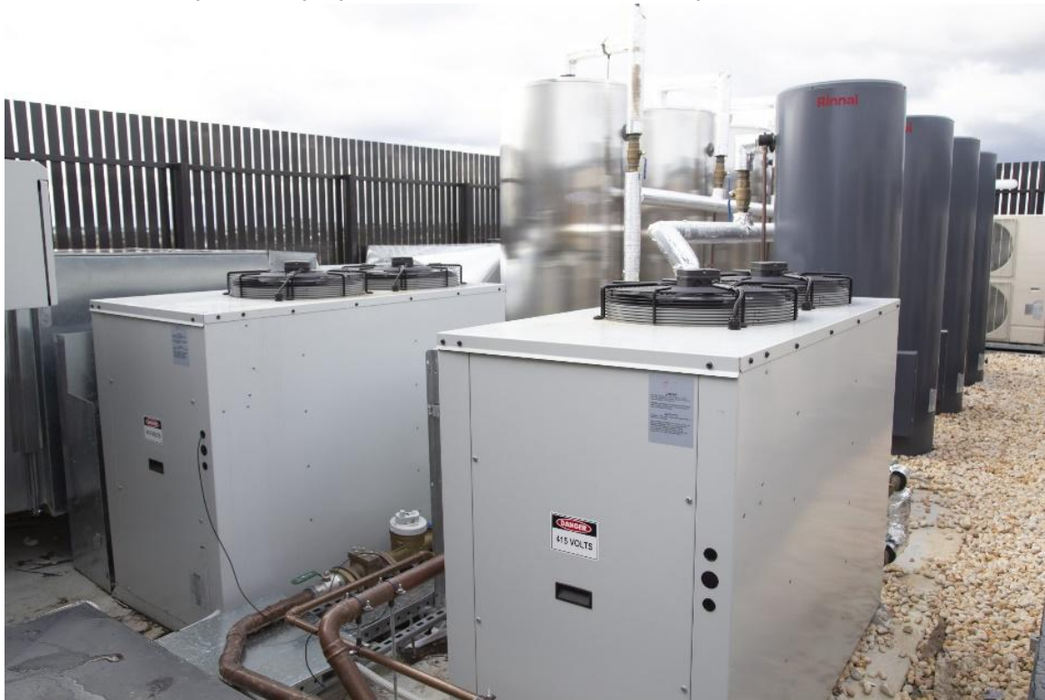
Figure 6- Typical heat pump set up
