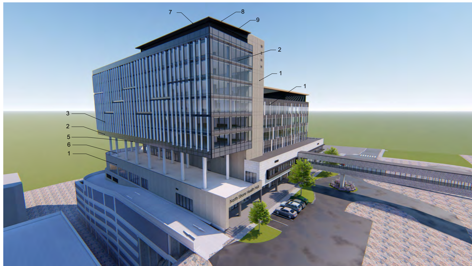
1. Vertical Shading aluminium powder coat white
